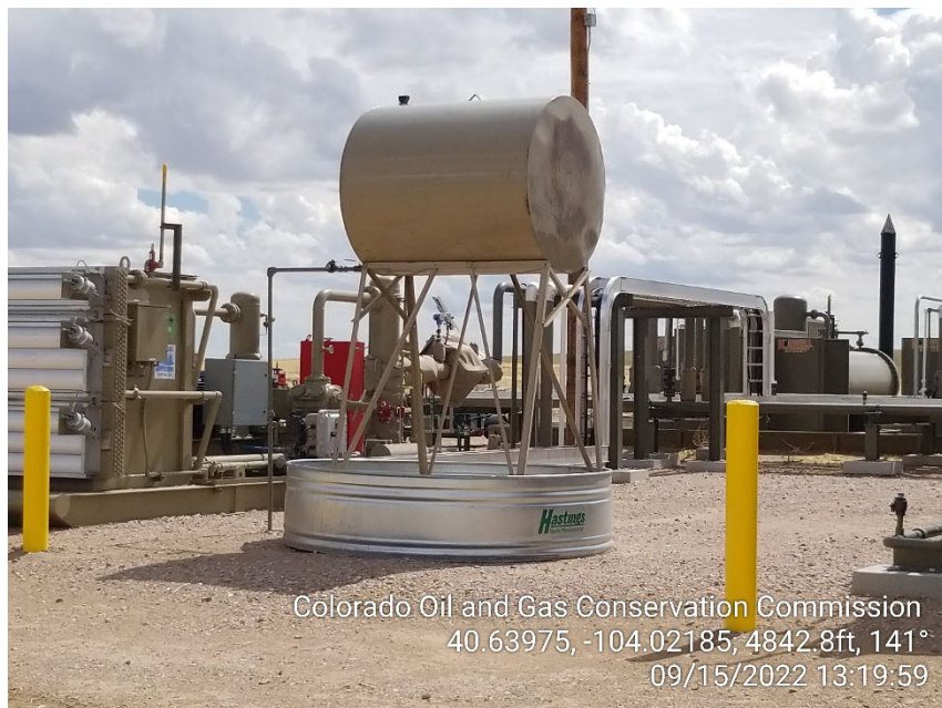
Photo 17 – Wildlife Netting missing on Day Tank
