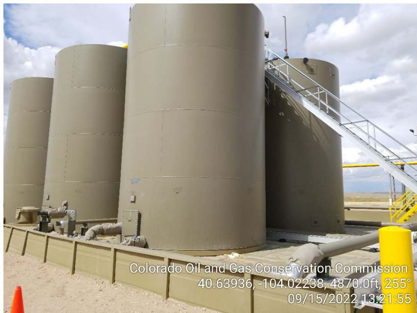
Photo 25 – Labels Missing on ALL Tanks
