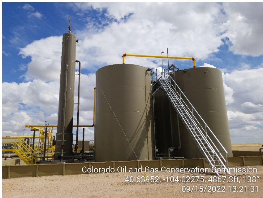
Photo 23 – VRT and Tanks – Labels Missing
