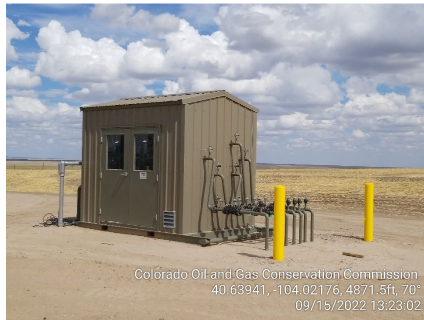
Photo 26 – Gas Lift Injection Meter House
