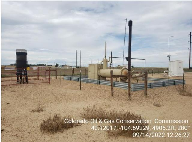
**Photo 13 ECD, HHS and gas Meter Run.**
