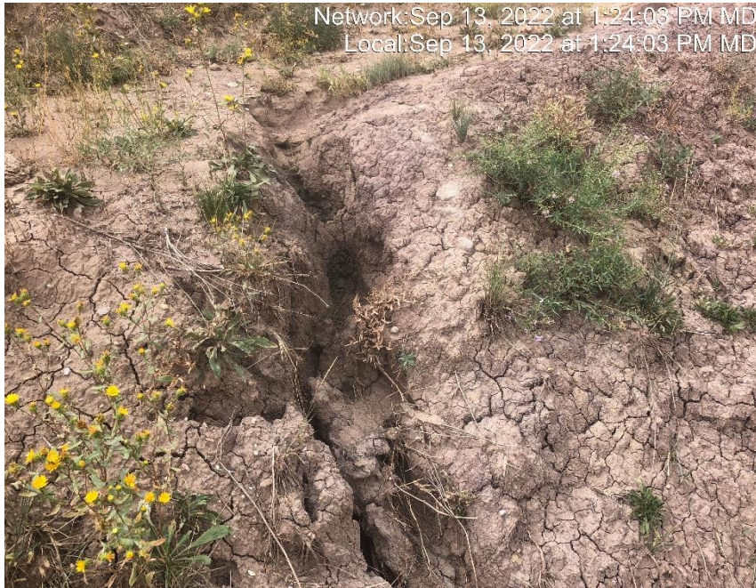
Photo #7662 Rill erosion occurring on cut slope.
