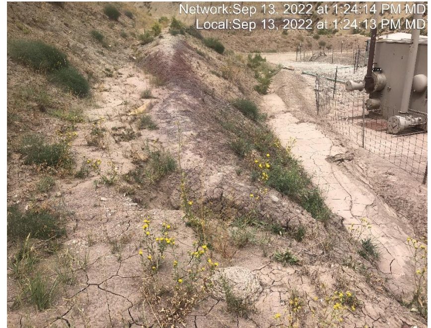
Photo #7663 Rill erosion occurring on cut slope.
