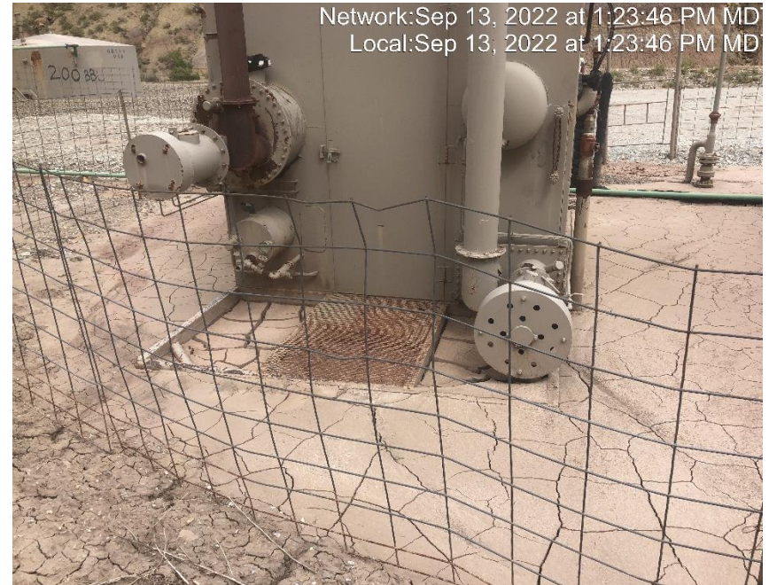
Photo #7661 Sediment is encroaching on equipment.
