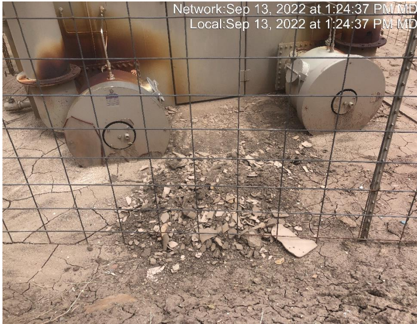
Photo #7665 Sediment encroaching on equipment.
