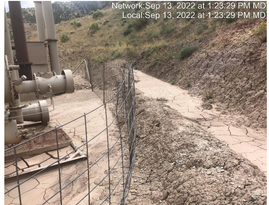
Photo #7659 Run on to location is not being controlled.
