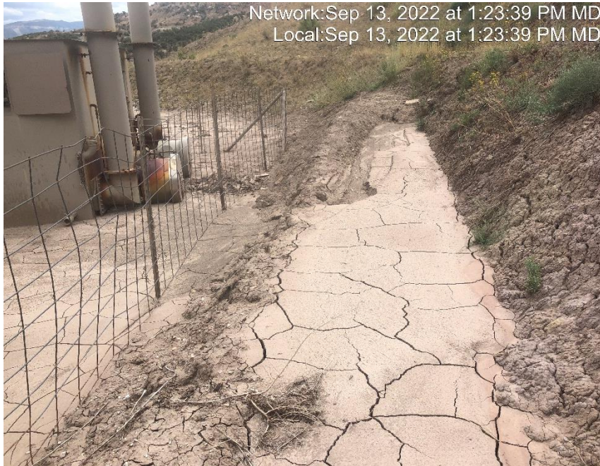
Photo #7660 Run on to location is not being controlled.
