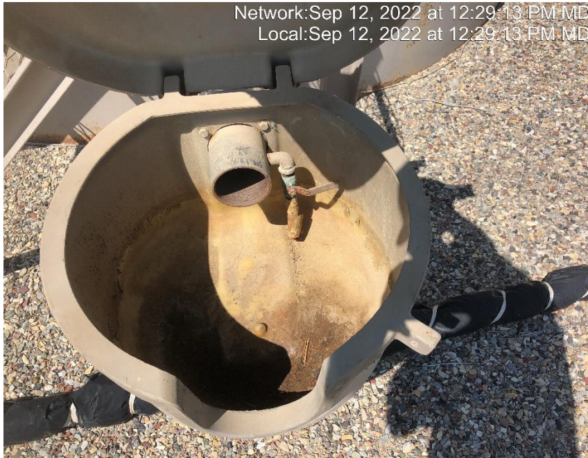
Photo #7634 Multiple loadlines open ended.
