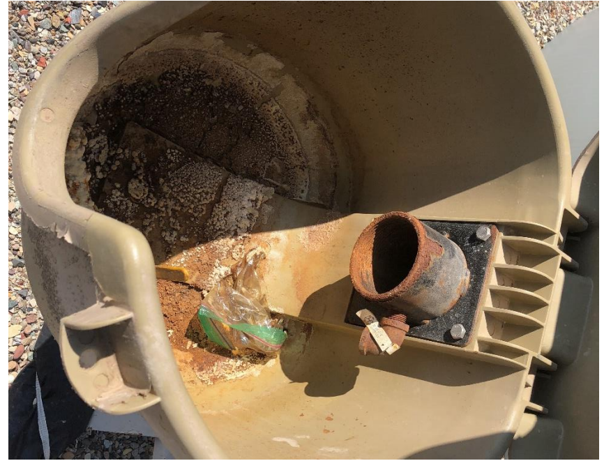
Photo #7635 Multiple loadlines open ended.
