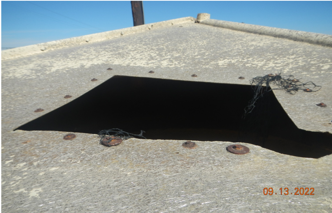
Photo 3. The netting at the top of the tank is inadequate.
