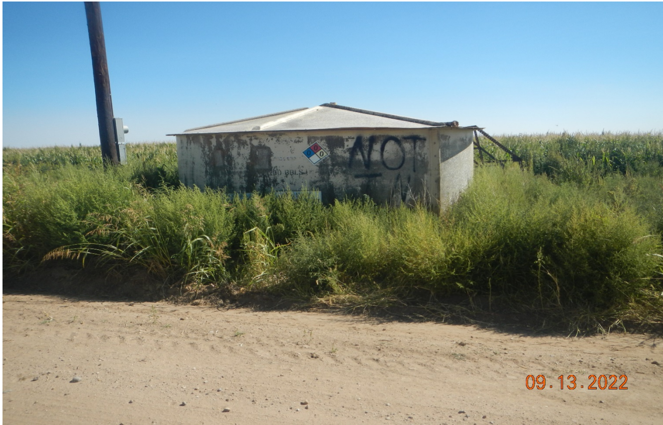
Photo 1. Facing east toward the tank battery along the access road. There is tall undesirable weeds around the tank that need to be removed. If take is not in use it must be removed. Tank berm is inadequate.
