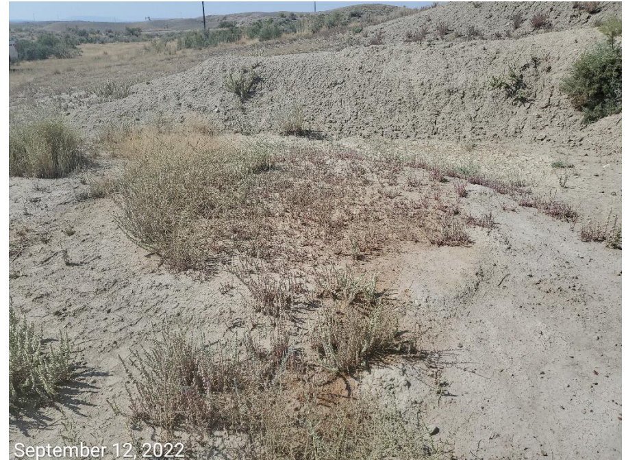
Photo 2: Photo shows remaining secondary containment berm; location has not been reclaimed.
