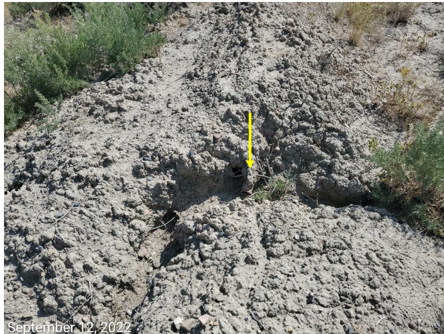
Photo 5: Photos taken from the north end of the Location. Photos show erosion degradation and partially buried unused pipe.
