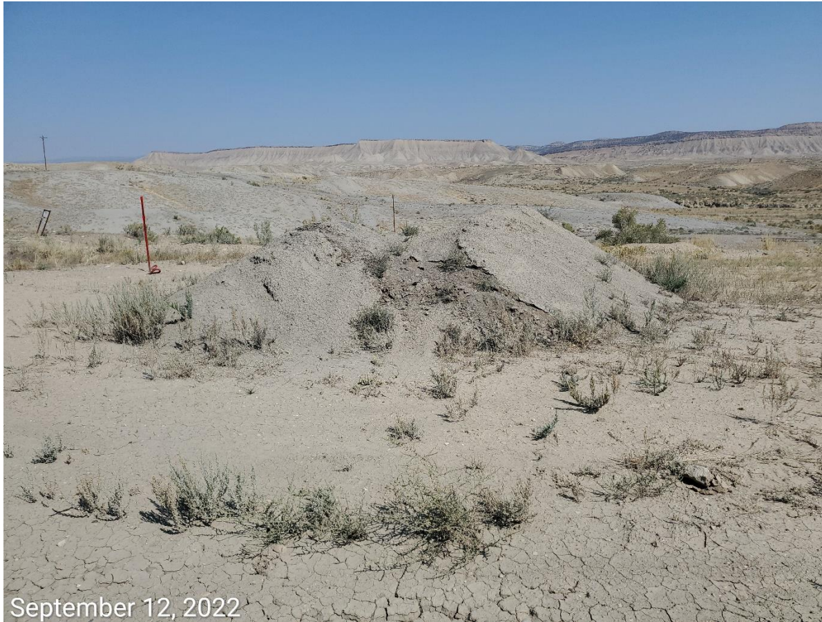
Photo 4: Topsoil stockpile on the north end of the Locaiton; stockpile missing BMPs per Rule 1002.c
