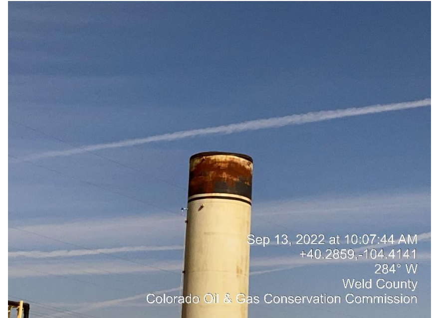
Photo #2 Bird protector appears to be missing
