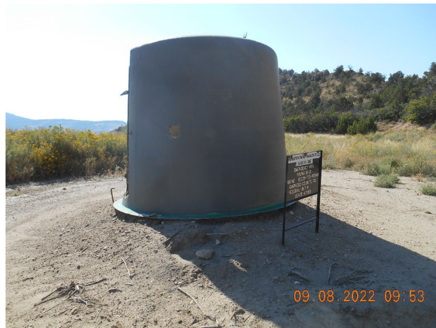
Wellhead inside fiberglass housing
