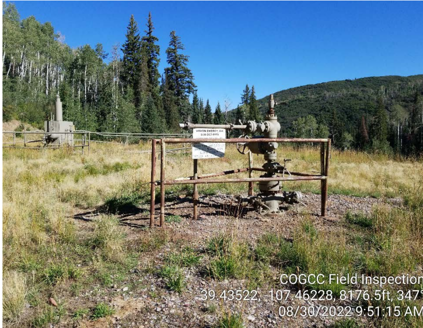
Photo #1 – Wellhead with sign, note horizontal separator in background.
