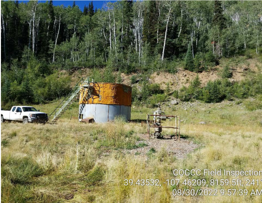
Photo #5 – View of wellhead and tank battery from east. This area was impacted by produced water reported under COGCC Spill/Release ID #482408.
