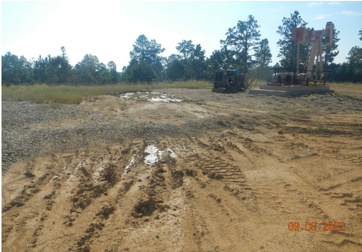
Photo 1. There is vehicle rutting and an area where is pooling at the location. This area needs to be repaired and stabilized.
