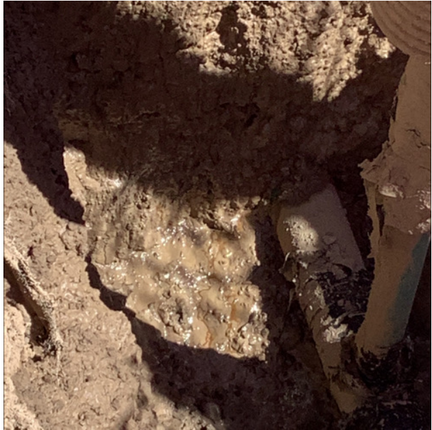
Fig. 12: All sidewalls within excavation appear discolored.
