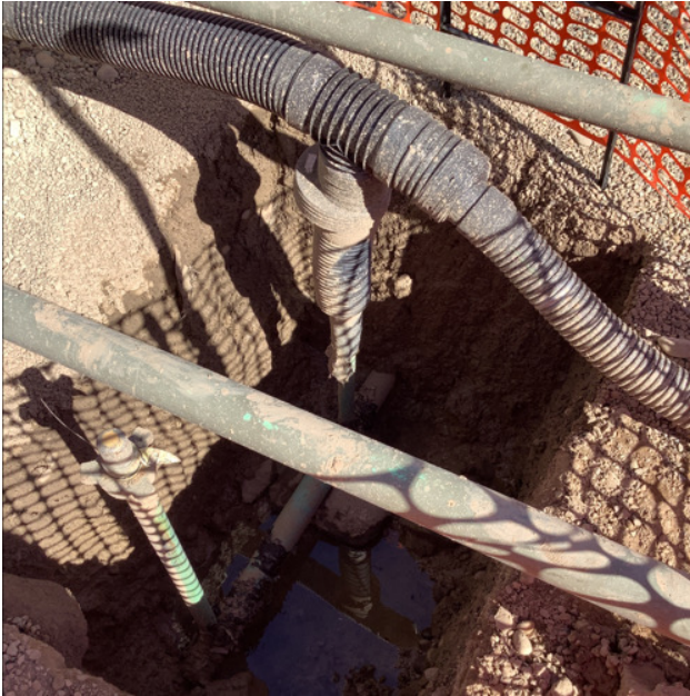
Fig. 11: Unknown water source pooled in base of excavation.
