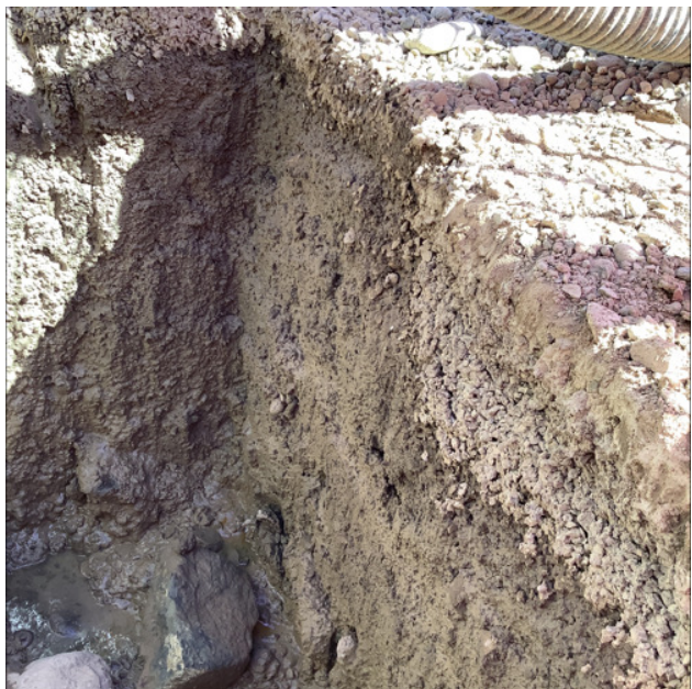
Fig. 12: All sidewalls within excavation appear discolored.
