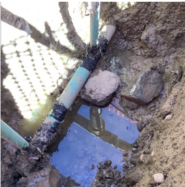
Fig. 11: Unknown water source pooled in base of excavation.
