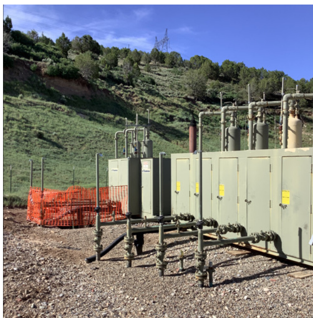
Fig. 8: Hydrovac excavation around south most separator unit. Orange safety net is around excavation.
