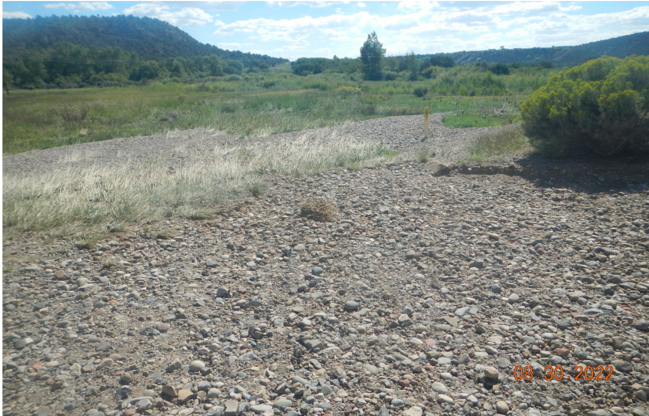
Photo 3. Facing southwest at the entrance of the location. Stormwater directed from the previous photo has washed gravel off the road onto the adjacent land.
