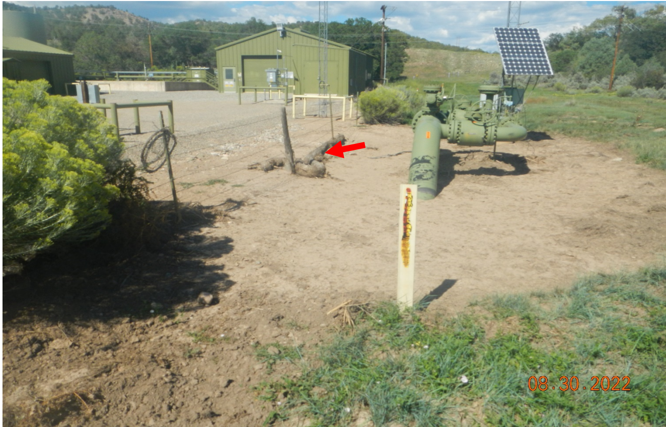
Photo 2. Facing northeast at the location. Stormwater had washed thru this area and displaced the wattles at the red arrow.
