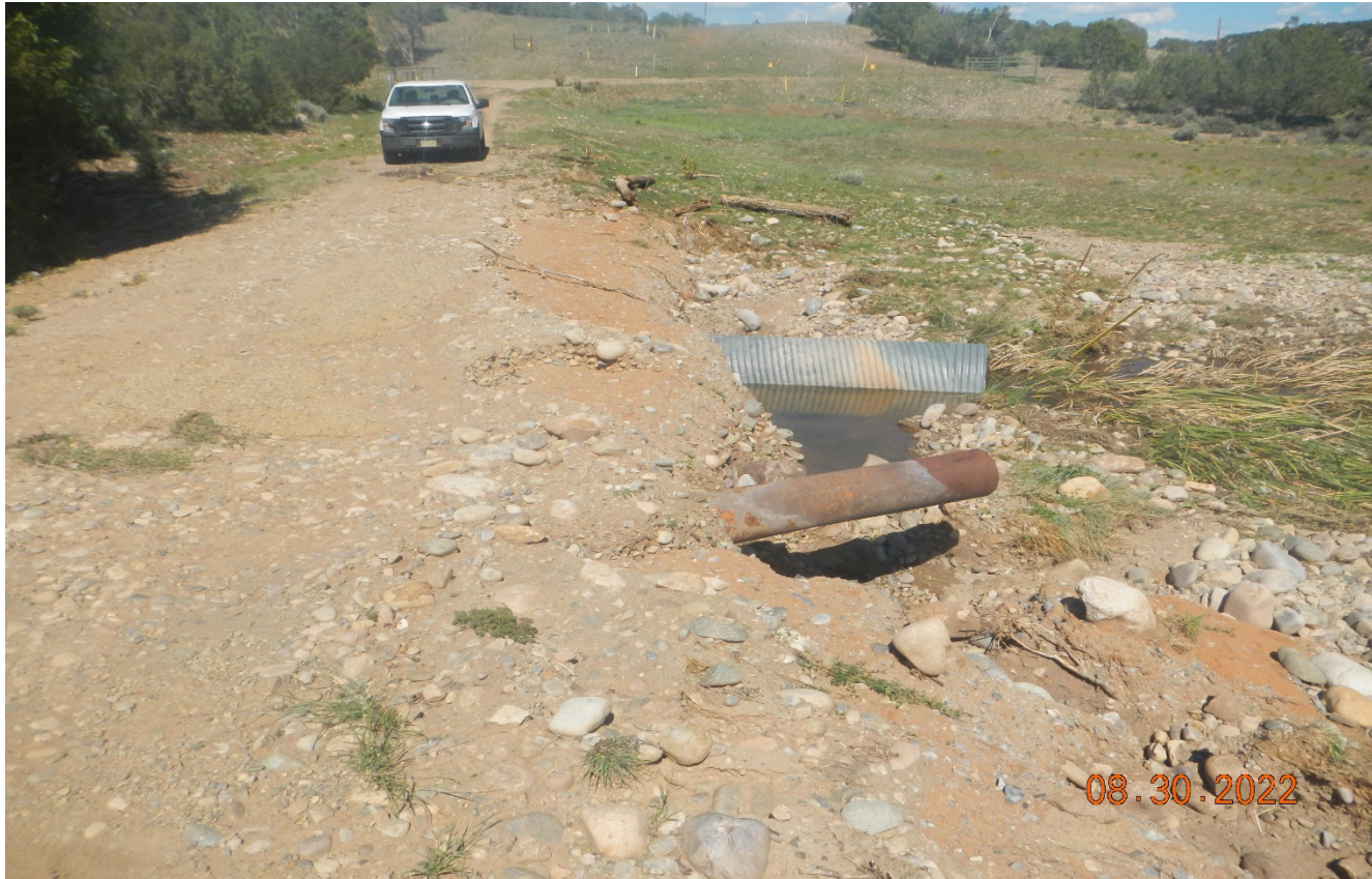
Photo 2. Facing back east along the access road. The road has been washed out in this area and will need to be repaired and stabilized.
