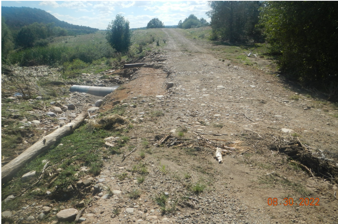
Photo 1. Facing west along the access road. The road has been washed out in this area and will need to be repaired and stabilized.
