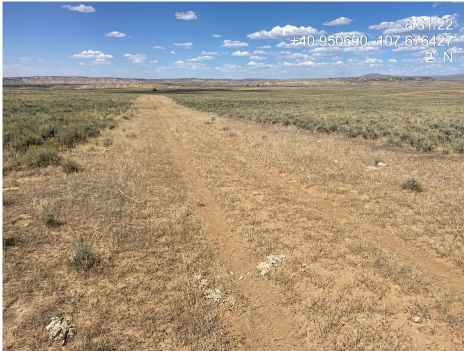
Photo 1. Photo taken to the north of the Location shows the access road remains. Vegetation growth is absent in tire tracks where soils are compacted and bare.
