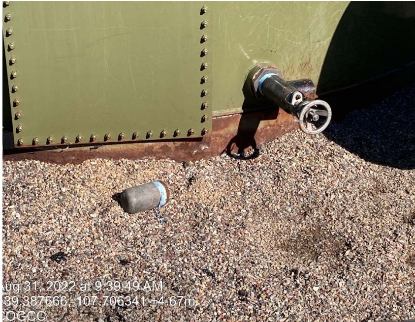
Valves missing plugs
