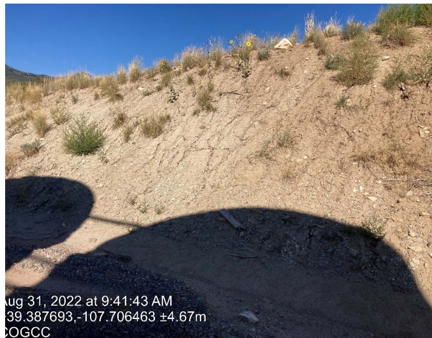
Cut slope erosion
