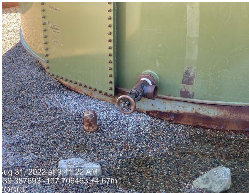
Valves missing plugs
