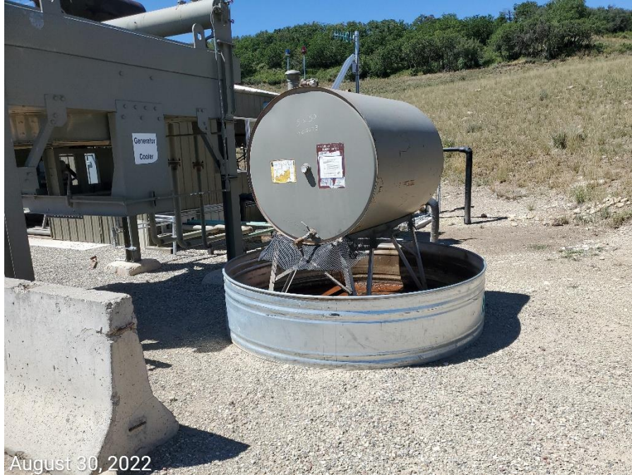
Photo 3: Photo shows tanks on the location with missing wildlife protection BMPs
