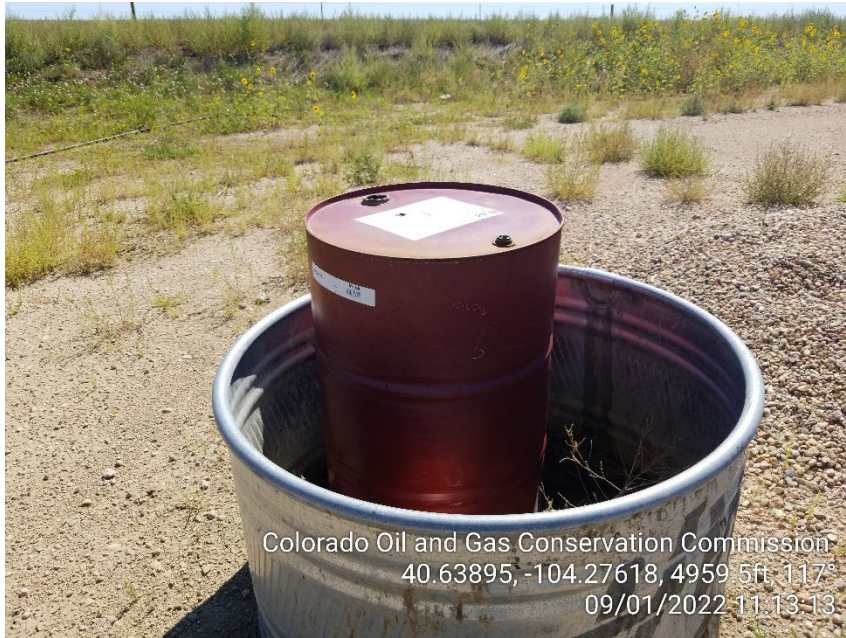
Photo 7 – Secondary Containment – Wildlife Netting missing
