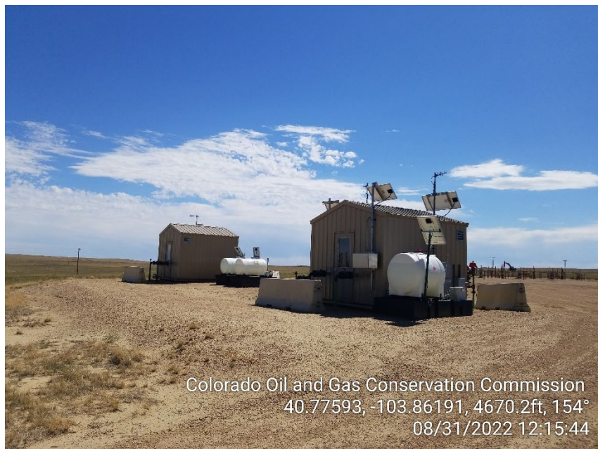
Photo 1 – Gas Lift Injection Meter Houses
