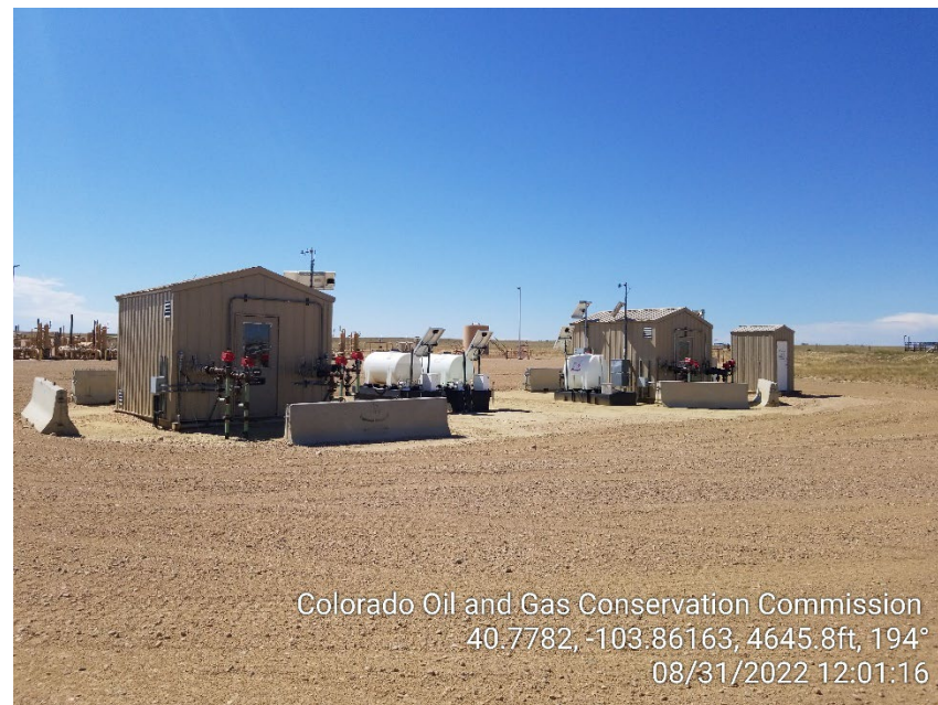
Photo 10 – Gas Lift Injection Meter Houses
