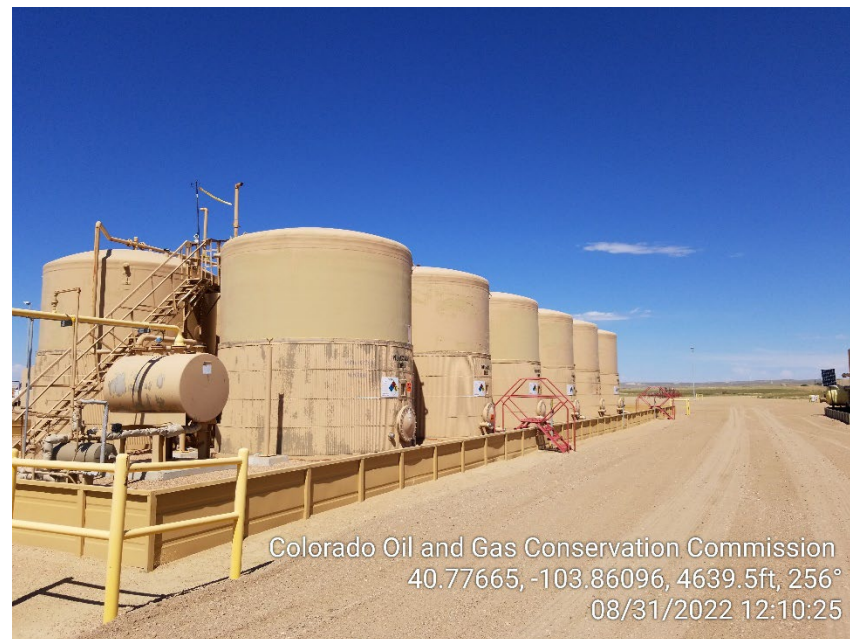
Photo 16 – Water Tank Battery
