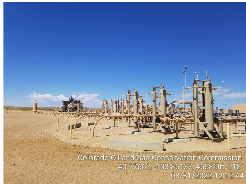
Photo 18 – Sand Traps and Headers
