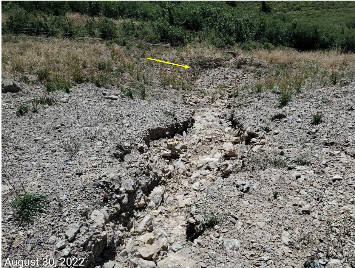
Photo 5: Continue from photo 4. Photo shows sediment trap (arrow). Photo shows outlet from the pad (inlet to the trap) has not been installed or maintained per good engineering practices, resulting in erosion (gully) degradation. Slopes require stabilization and additional reclamation.
