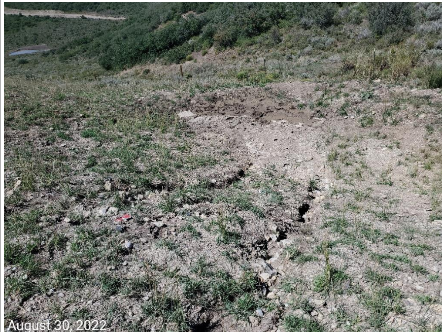
Photo 11: Photo taken from the sediment trap on the north end of the Location, adjacent to the Location entrance; BMP has not been installed or maintained per good engineering practices, resulting in degradation at the inlet and outlet of the control.
