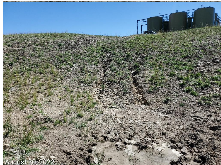
Photo 11: Photo taken from the sediment trap on the north end of the Location, adjacent to the Location entrance; BMP has not been installed or maintained per good engineering practices, resulting in degradation at the inlet and outlet of the control.
