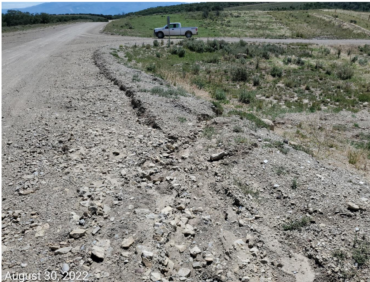
Photo 12: Photo taken from the main access road north of the Location (~ 39.500266/-108.182963). Photo shows stormwater runoff has resulted erosion degradation at the slope, and sediment transport/deposition.
