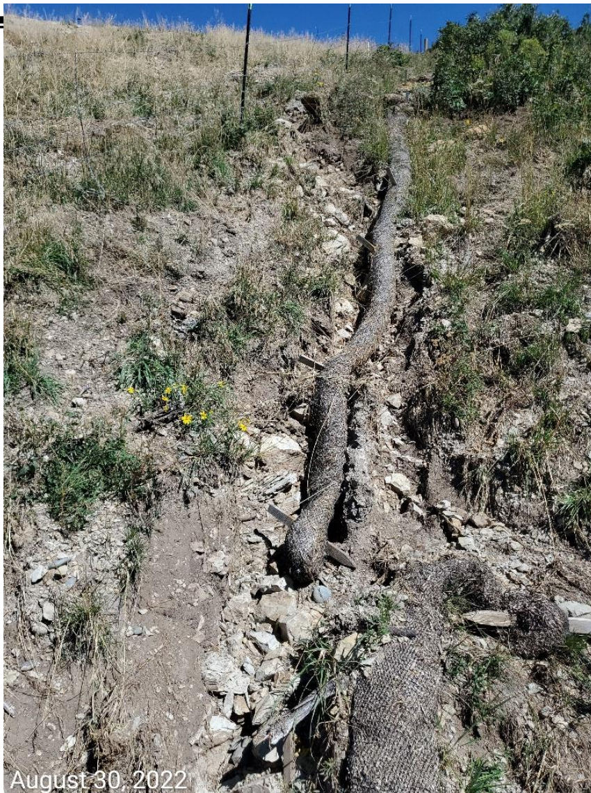
Photo 9: Continued from photo 8. Photo shows off-site areas below the eastern sediment trap, and the Location; BMPs to manage runoff in such a manner as to minimize erosion, degradation and offsite sediment transport are inadequate. Disturbed areas require stabilization and reclamation.
