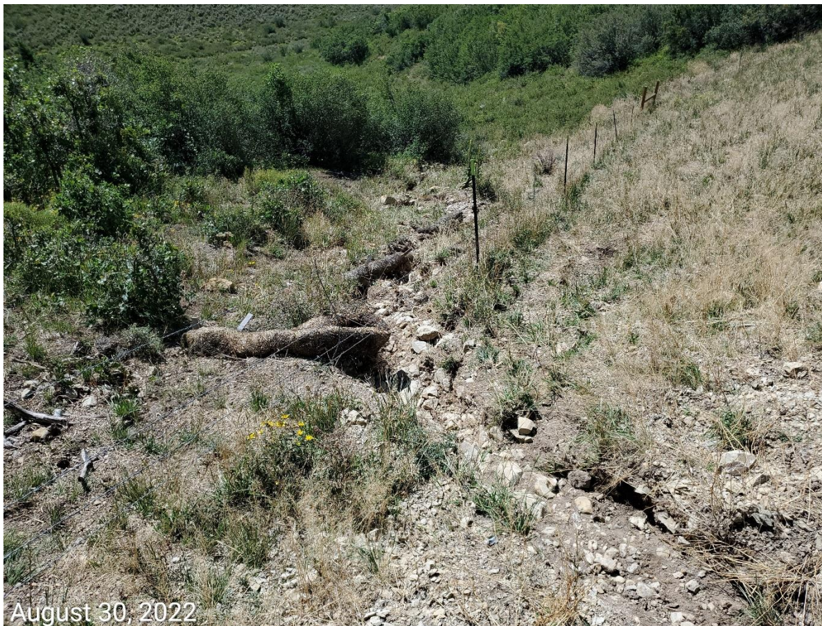
Photo 8: Photo shows off-site areas below the sediment trap on the east end of the Location; BMPs to manage runoff in such a manner as to minimize erosion, degradation and offsite sediment transport are inadequate. Photo also shows erosion logs along the perimeter have not been maintained, and are considered “debris”. Fence in photo is the edge of the Location’s disturbance area. Disturbed areas require stabilization and reclamation.
