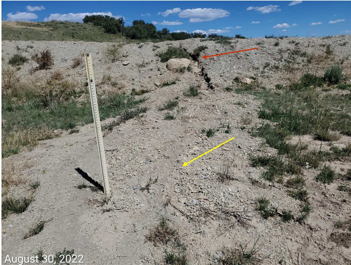
Photo 13: Continued from photo 12. Photo shows Stormwater runoff from the main access road north of the Location has resulted in gully erosion (red arrow) and sediment transport/deposition (yellow arrow).
