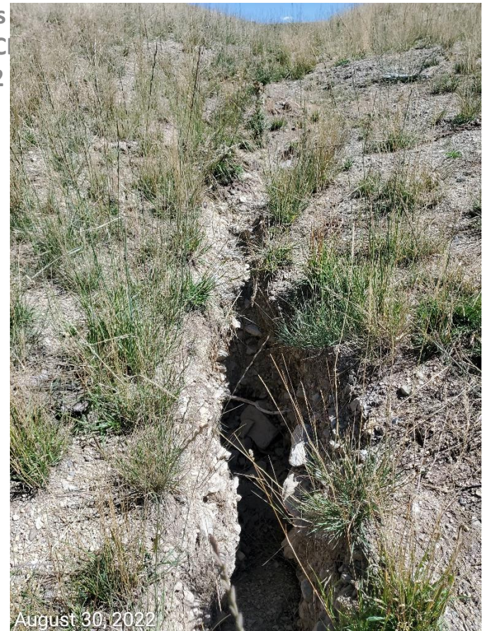
Photo 5: Photos taken from the sediment trap on the southwest end of the Location. Photo shows gulley erosion at inlet of the trap.
