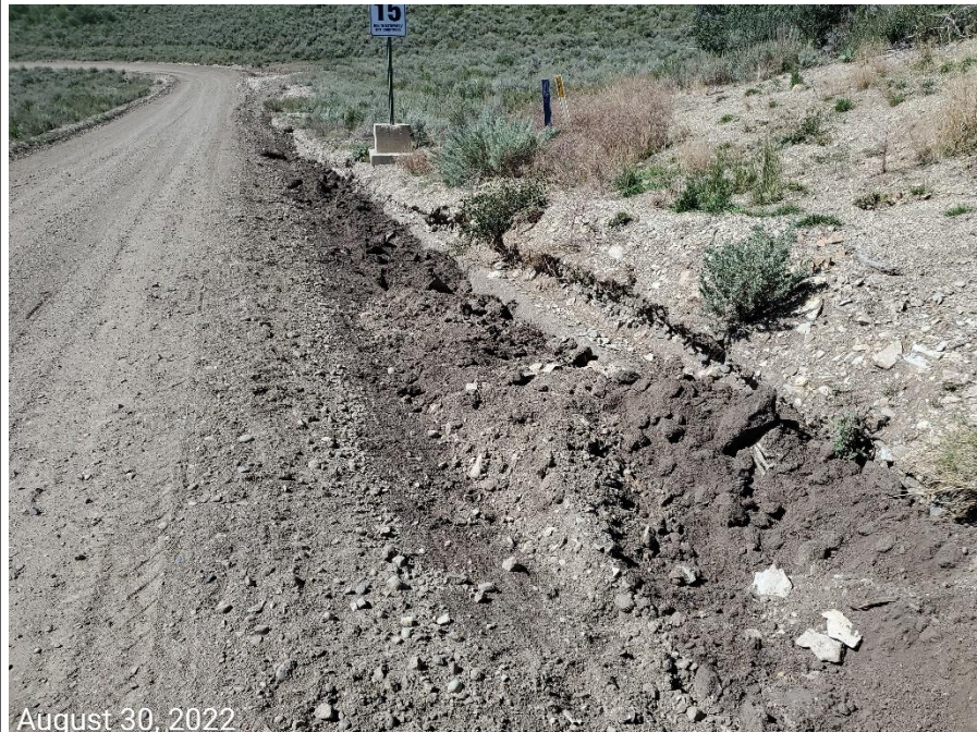
Photo 6: Photos taken from the access road. Photos examples showing erosion degradation evident at the stormwater diversion ditch; additional unconsolidated soils also appear to have been put into the ditch; this will contribute to sediment-laden stormwater discharge.
