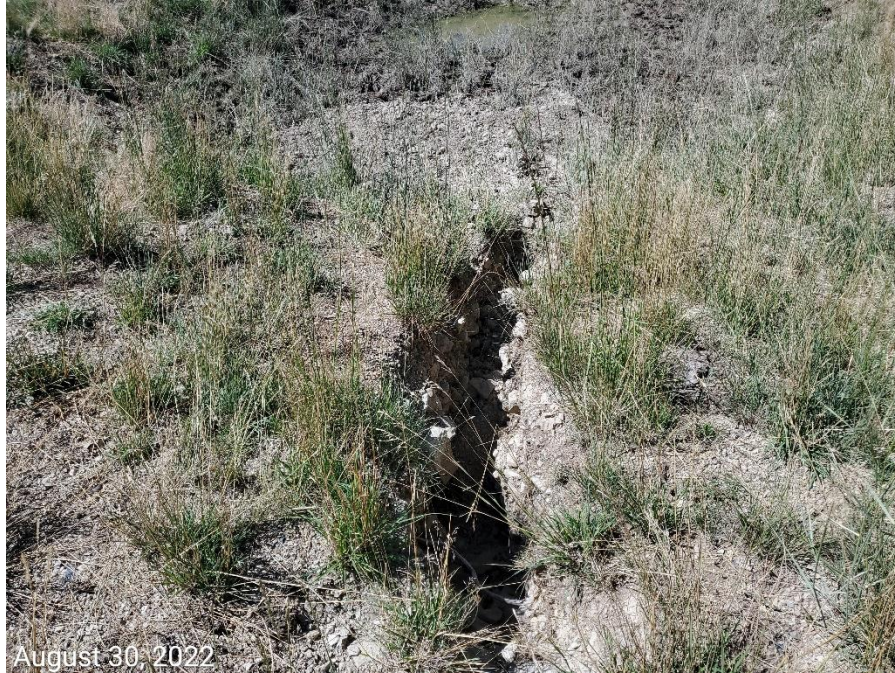
Photo 5: Photos taken from the sediment trap on the southwest end of the Location. Photo shows gulley erosion at inlet of the trap.
