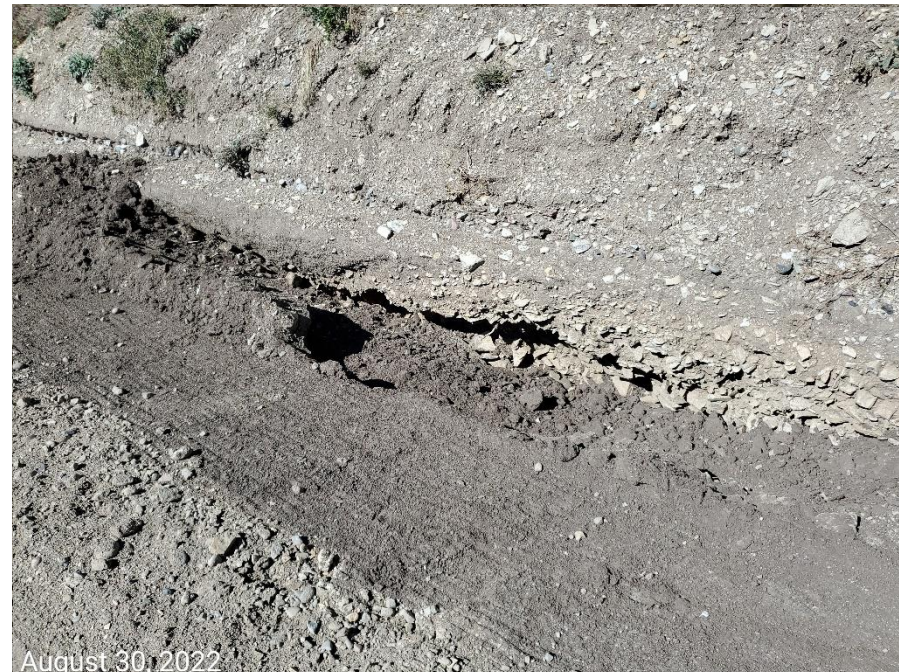
Photo 6: Photos taken from the access road. Photos examples showing erosion degradation evident at the stormwater diversion ditch; additional unconsolidated soils also appear to have been put into the ditch; this will contribute to sediment-laden stormwater discharge.
