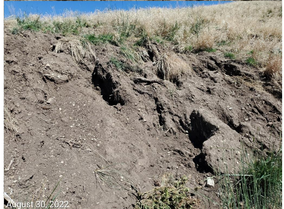
Photo 4: Photo taken from the sediment trap on the southwest end of the Location; photo shows erosion degradation observed on the south facing slopes.
