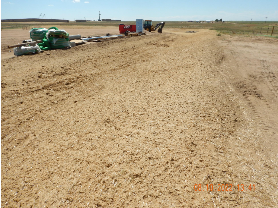
Photo 3. Photo taken from the northeastern location, facing West. Photo illustrates the eastern sediment basin area which has been seeded, straw crimped with mulch and tackifier applied.
