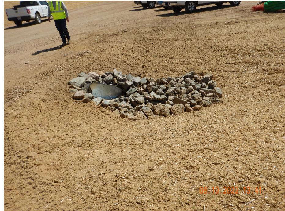
Photo 2. Photo taken from the entrance of location, facing South. Photo illustrates the stabilized outlet of the culvert which is directed to a sediment basin.
