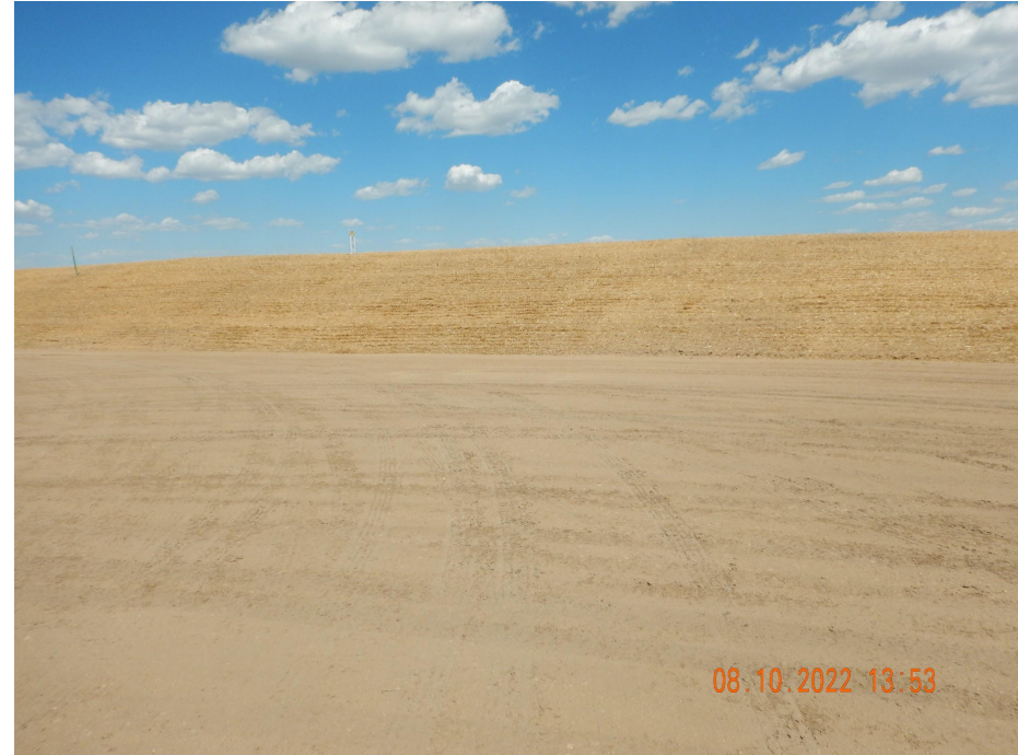
Photo 8. Photo taken from the eastern location, facing East. Photo illustrates the topsoil stockpile which has been stabilized with seeding, straw crimped with mulch and tackifier applied.
