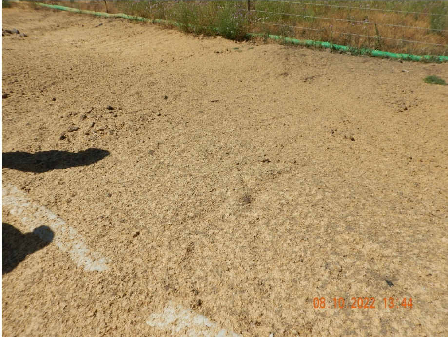
Photo 5. Photo taken from the weir of the outlet structure, facing Northwest. Photo illustrates the riprap material has been buried.
