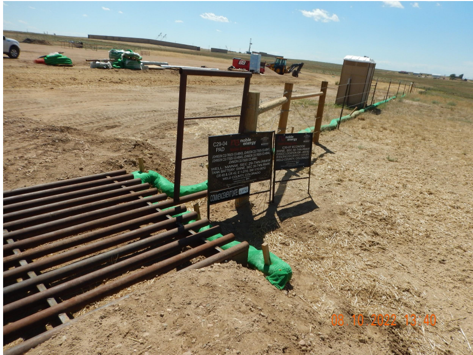
Photo 1. Photo taken from the entrance of location, facing Southwest. Photo illustrates a cattle guard which would also serve as a VTC device BMP. Also, filtrex has been installed around the entire perimeter of location.
