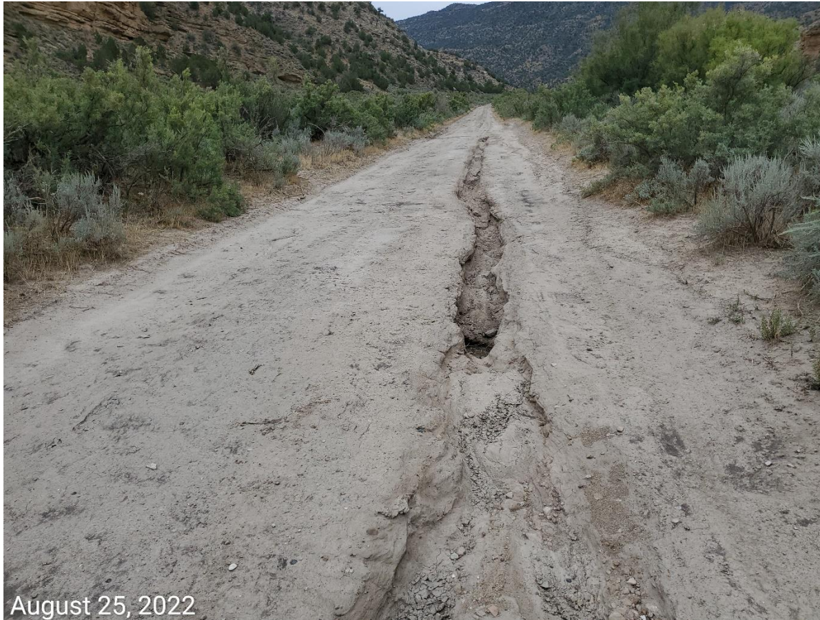
Photo 10: Photo taken from the access road south of Utah Gas Corp's Federal-Carbonera 1-2; access road is shared between the two Operators. Photo shows erosion control and stabilization BMPs are missing or insufficient along entire access road- erosion degradation and sediment transport evident.
