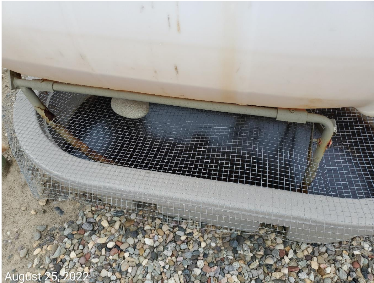
Photo 6: Continue from photo 5. Photo show fluids within the secondary containment of the methanol tank.
