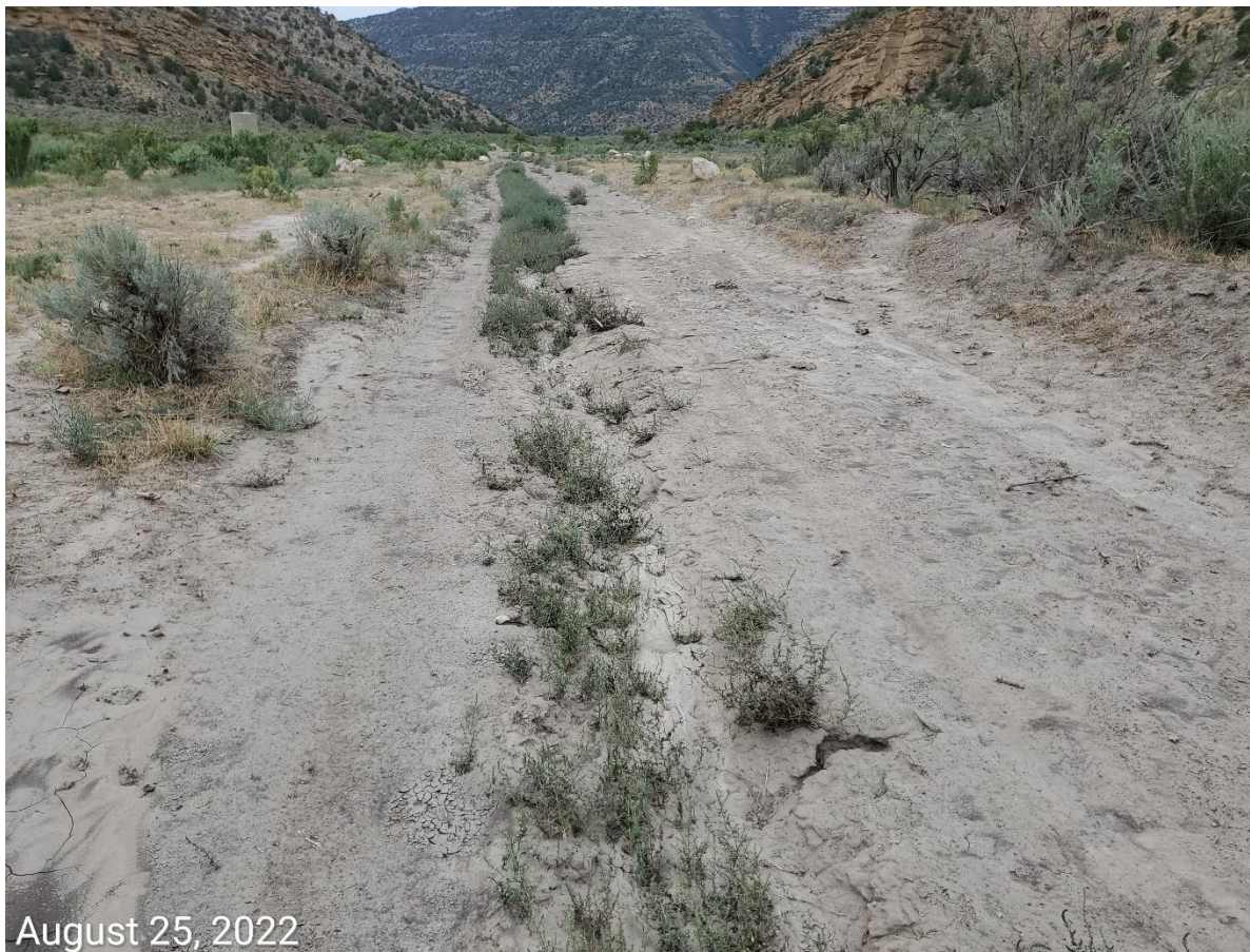
Photo 9: Photo taken from the access road between Utah Gas Corp's Federal-Carbonera 1-2, and Locin's Government 1 Location; access road is shared between the two Operators. Photo shows erosion control and stabilization BMPs are missing or insufficient along entire access road- erosion degradation and sediment transport evident.
