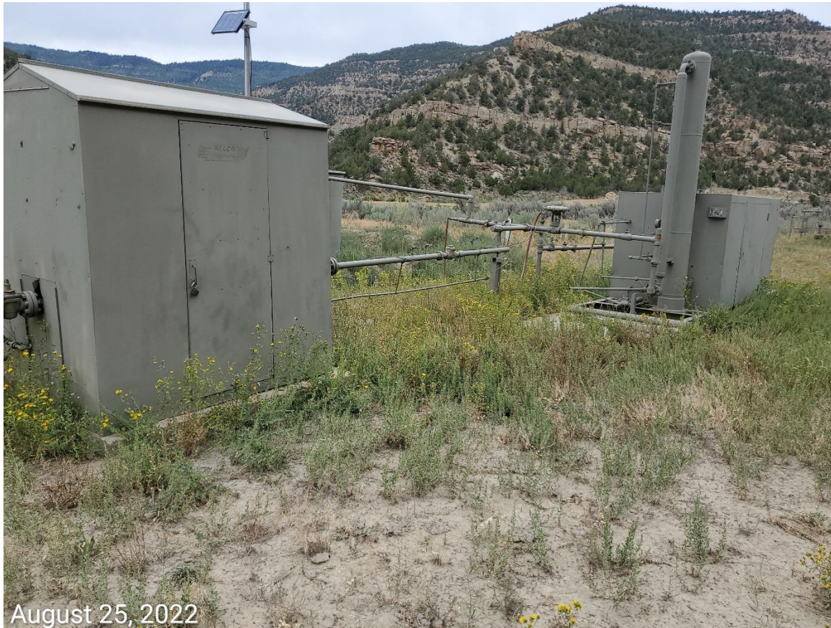
Photo 6: Photo shows weeds have re-established at and around production equipment on the Location; this is a fire hazard
