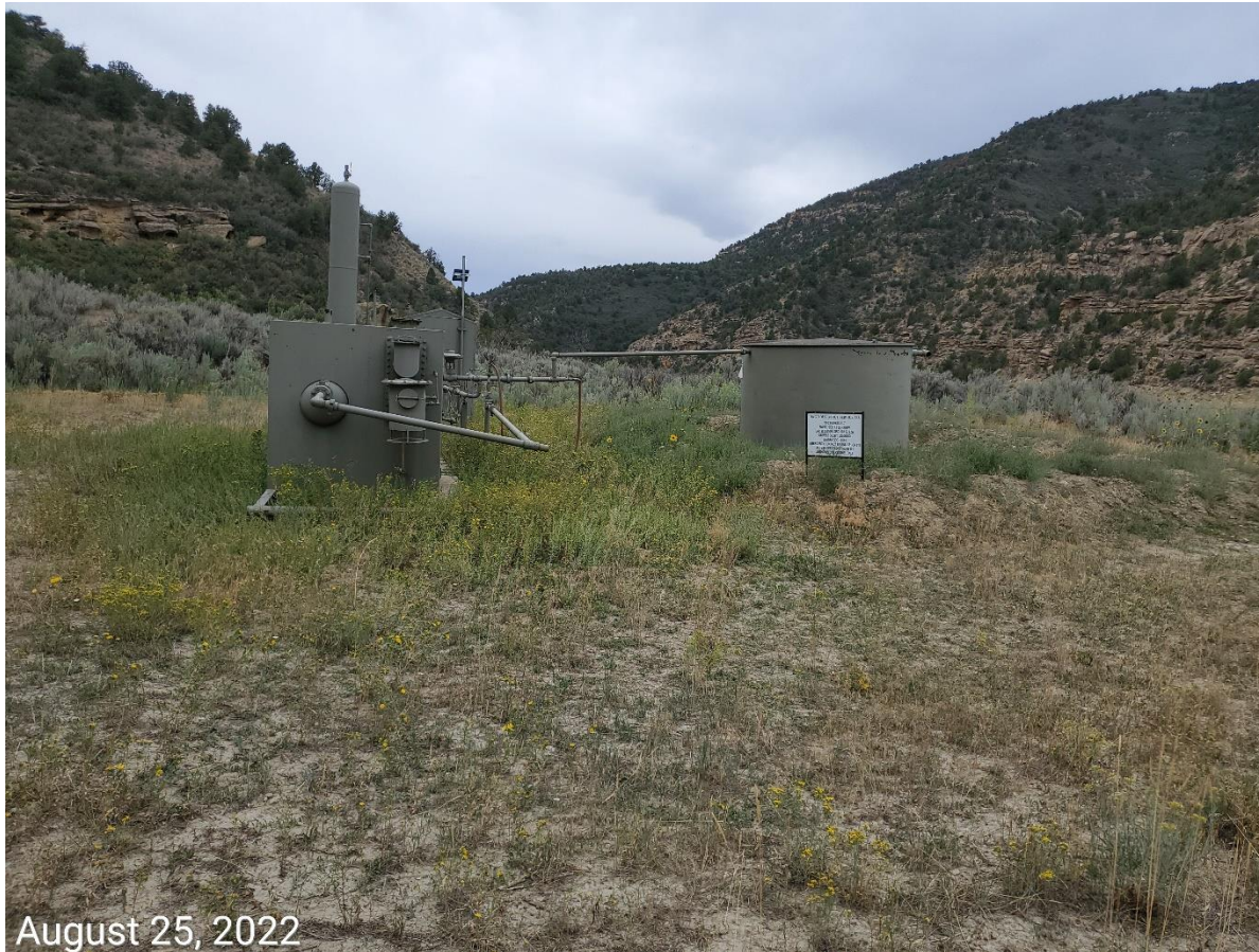
Photo 3: Photo shows weeds have re-established at and around production equipment on the Location; this is a fire hazard
