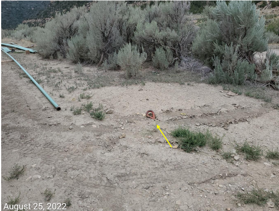
Photo 3: Northwestern anchor missing required marking.
