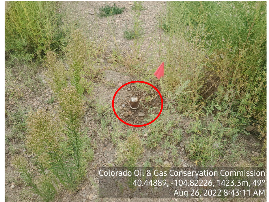
Photo 6: Marked riser to be removed
