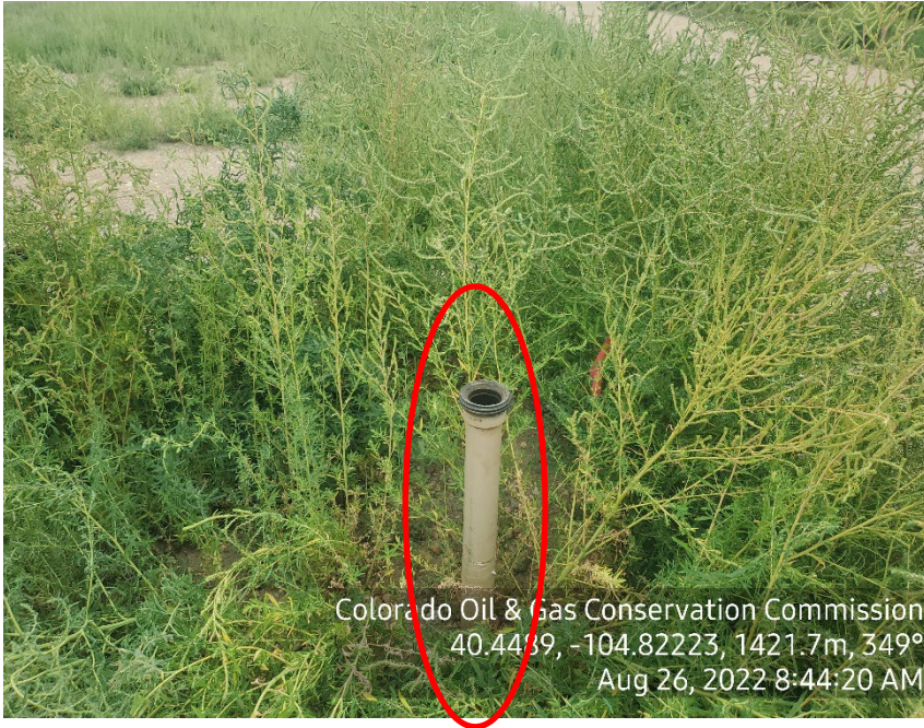
Photo 9: Marked riser to be removed
