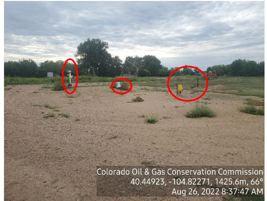
Photo 4: Production equipment removed, risers remain
