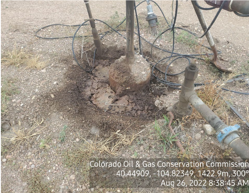
Photo 3: Stained soil at pumpjack
