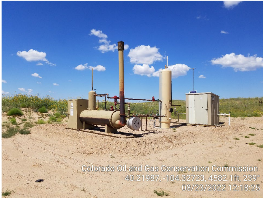
Photo 3 – Separator and Gas Meter
