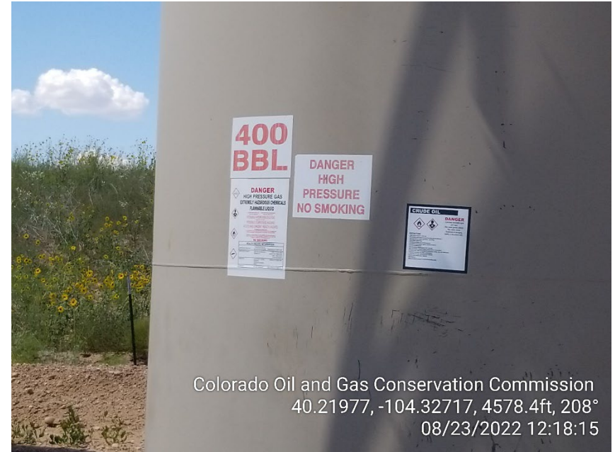
Photo 2 – Tank Labels – NFPA Label missing
