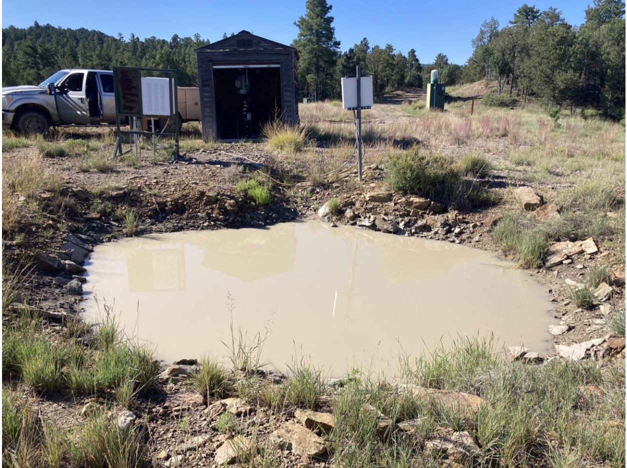
Lowered fluid level so at least two feet of freeboard exists per Rule 909.c
