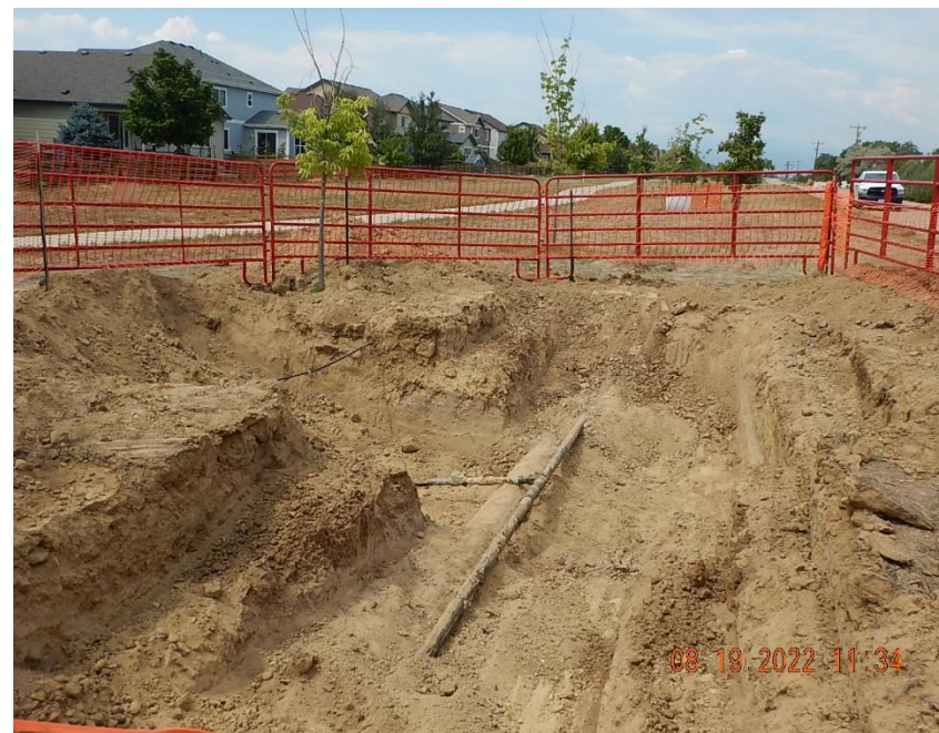
View of flowlines exposed in east bellhole excavation during repairs; view W along WCR 14.5
