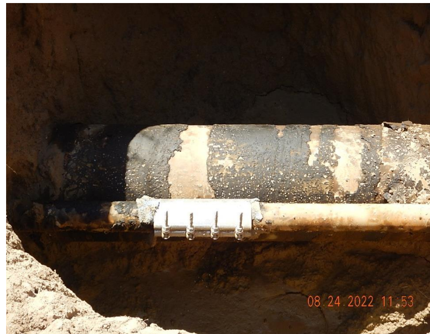
View of flowlines exposed in excavation at release point; (1) 4" carbon steel flowline (being repaired) with a bolted clamp over hole in line; (1) 16"-18" CS OLF (consolidation).
