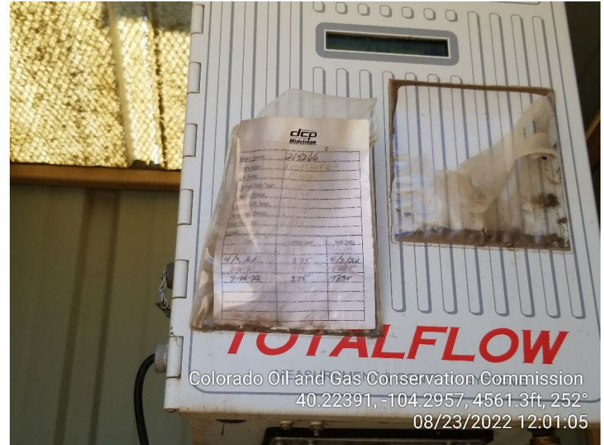
Photo 6 – Gas Meter Calibration Card
