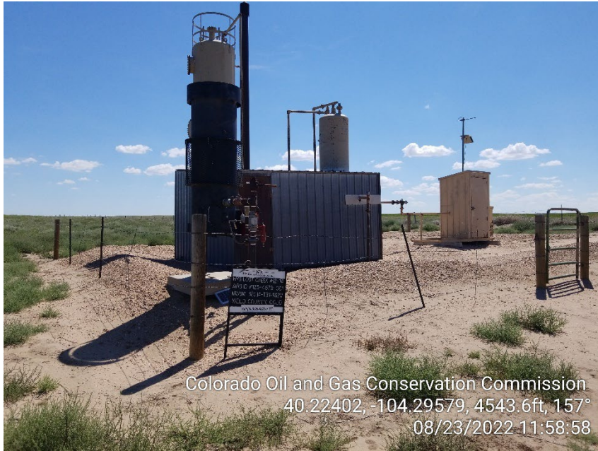
Photo 5 – Heater Treater and Gas Meter
