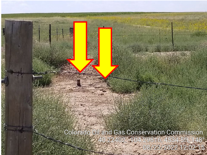
Photo 9 – Unmarked Risers
