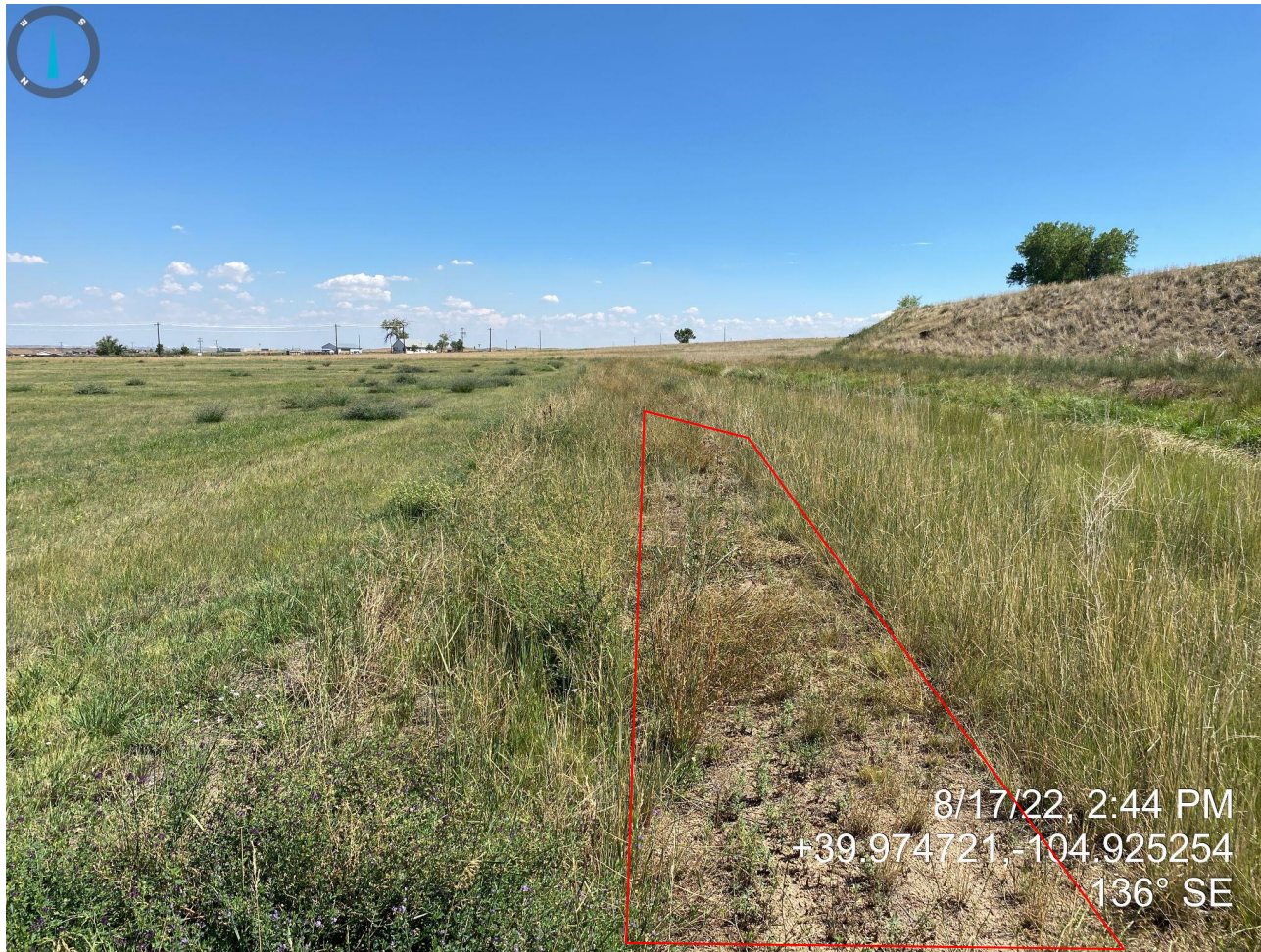
Photo 13. Access road photo taken south of location, facing southeast. Photo illustrates some desirable vegetation along portions of the access road; gravel/road base observed within new growth (highlighted in red).
