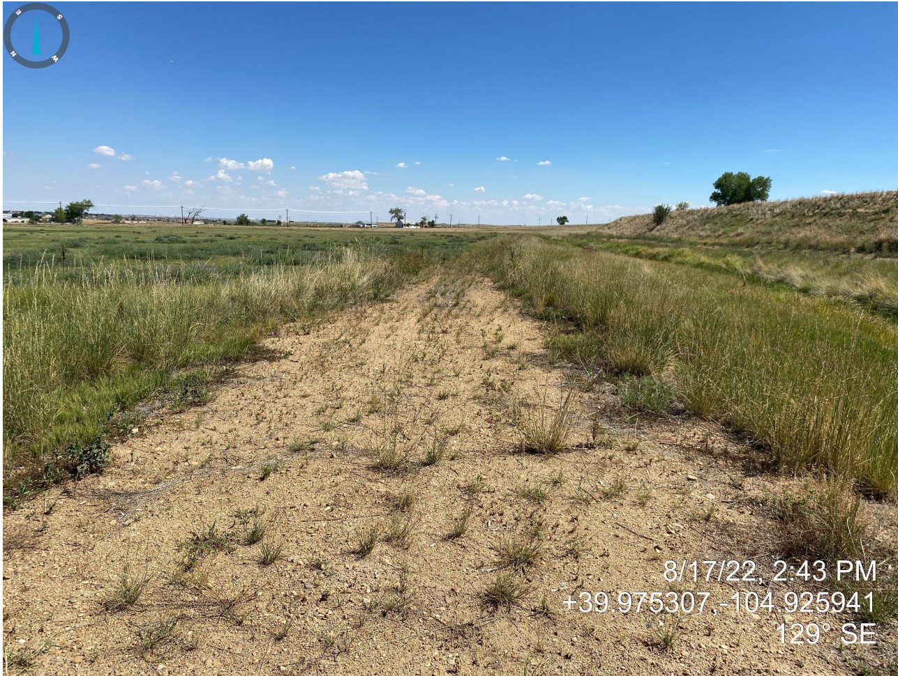
Photo 11. Access road photo taken south of location, facing southeast. Photo illustrates access road has not been reclaimed with presence of gravel/road base.
