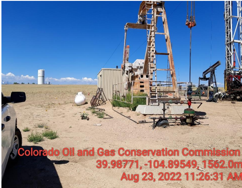
Photo 1 Stained soil around well head. Unused equipment (pipe and fencing). Weeds around equipment
