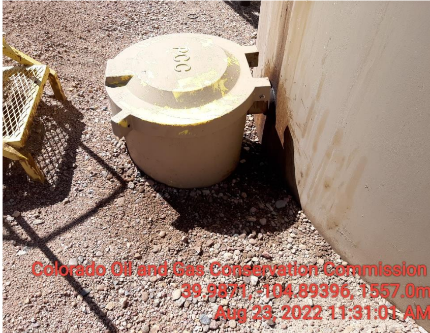
Photo 9 Stained soil around crude oil loadout line
