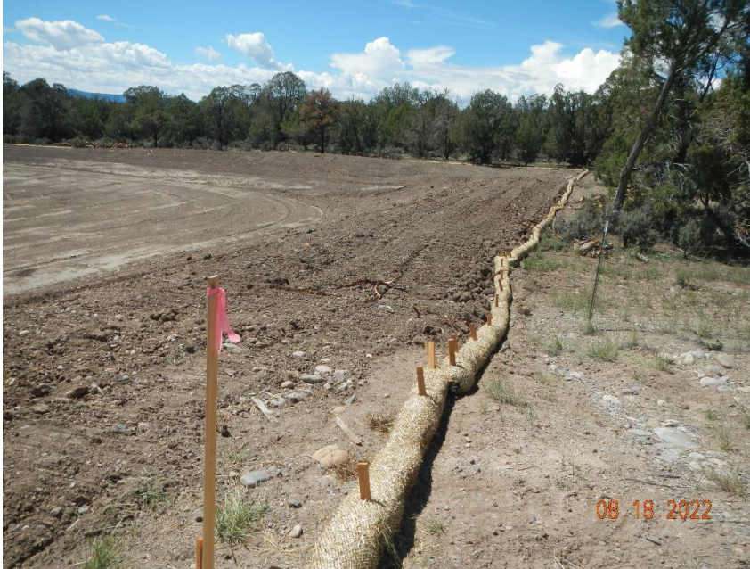
Wattle installation on south side of disturbance
