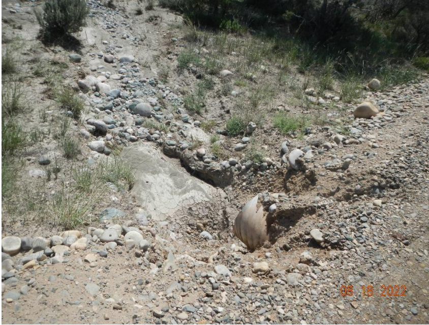
Erosion at culvert outlet on access
