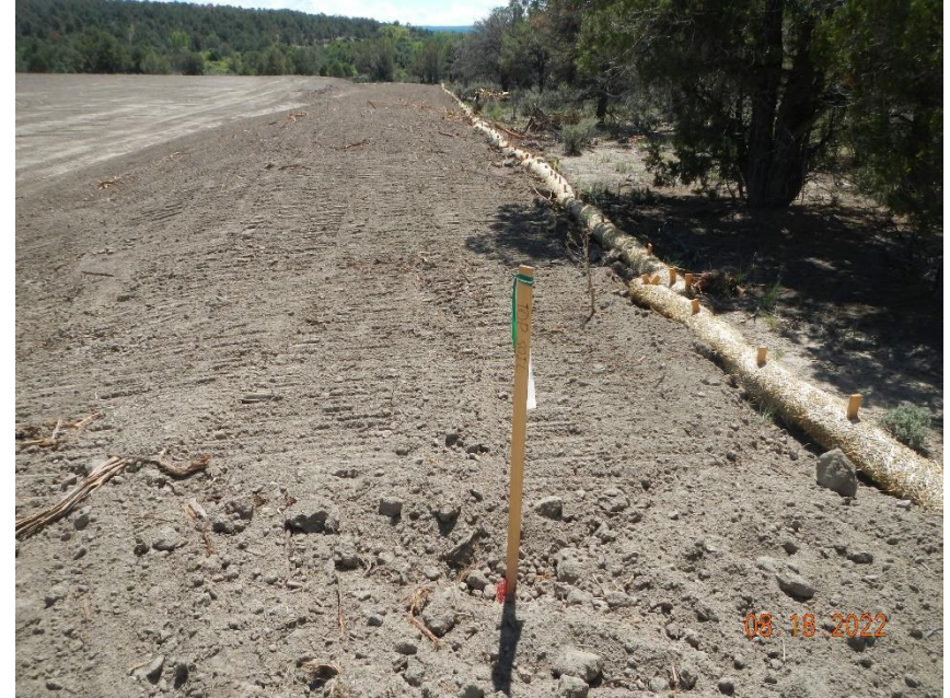
Stake in NE corner labeled “top soil” and what appears to be top soil storage in a board flattened area on perimeter of new disturbance arewa
