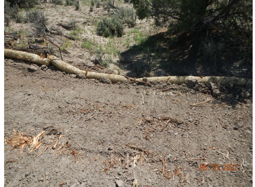
BMPs installation appears inadequate to control run-off on south side of new disturbance
