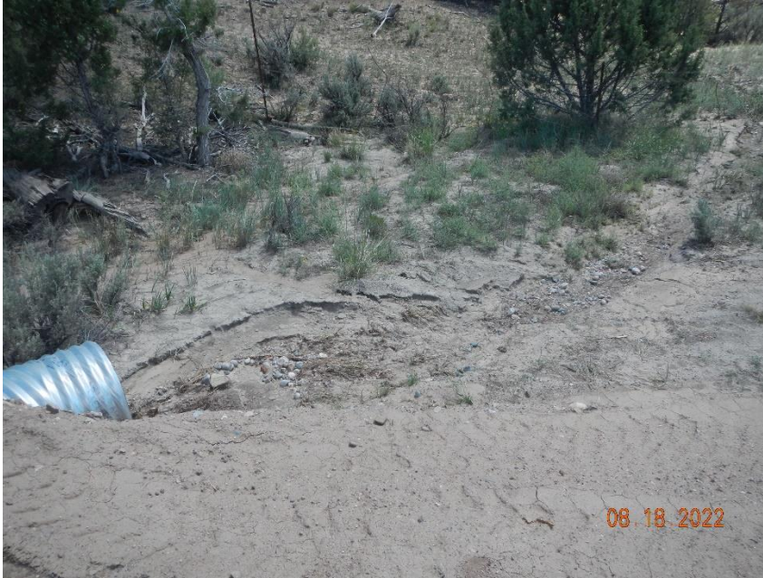
Stormwater erosion at culvert on access road, no outlet protection BMPs
