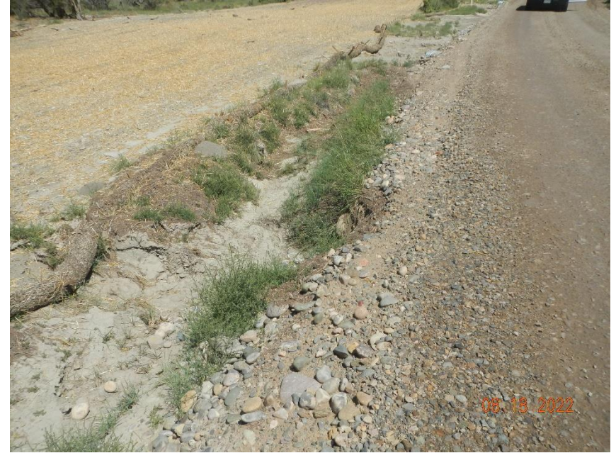
Erosion along access and improperly installed/maintained straw wattles
