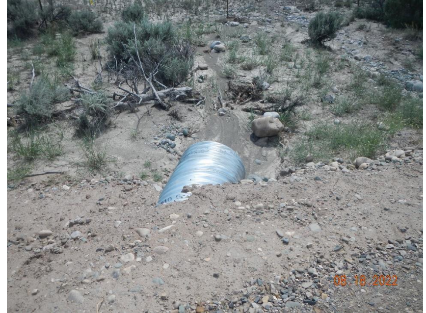
Erosion at culvert outlet on access
