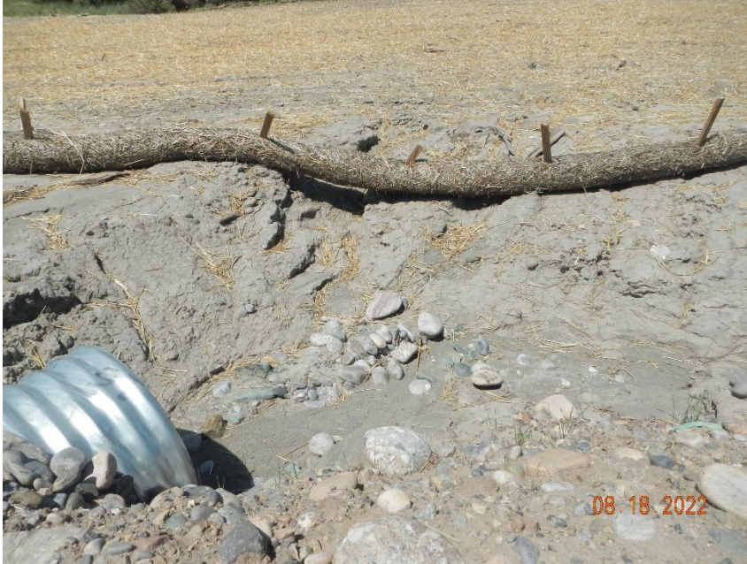
Erosion at culvert inlet on access road, improperly installed/maintained straw wattles
