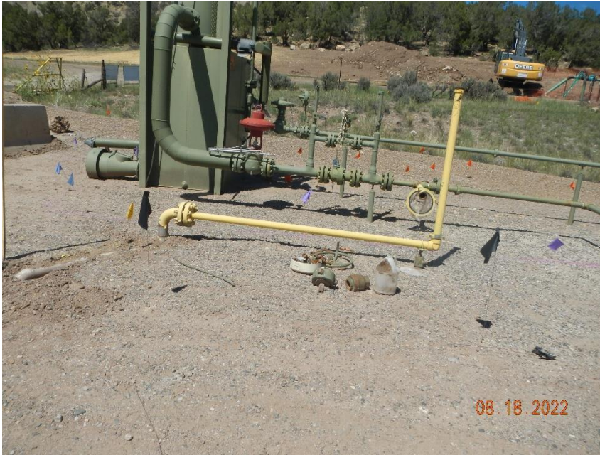
Production equipment from PA well not removed, unused parts
