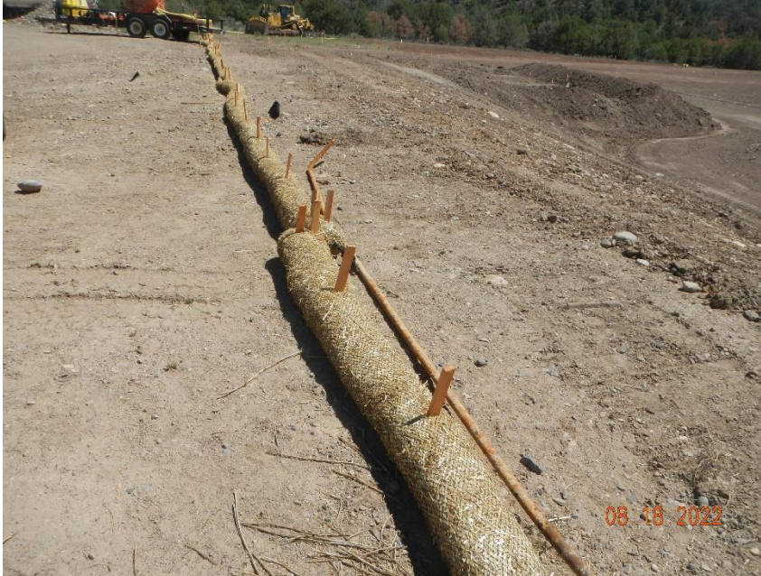
Vertically staked wattles, not trenched in on north side of new disturbance
