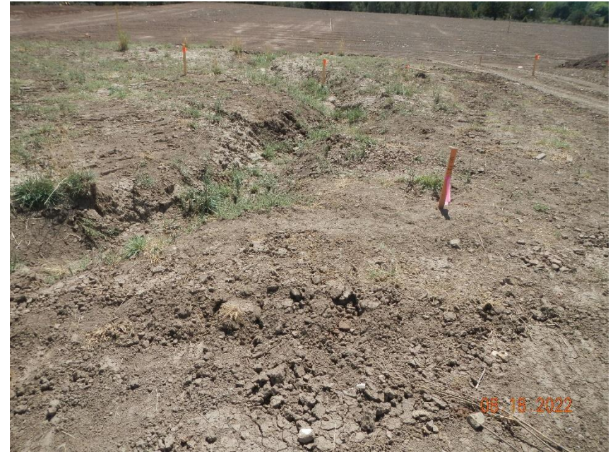
Erosion channel with no BMPs
