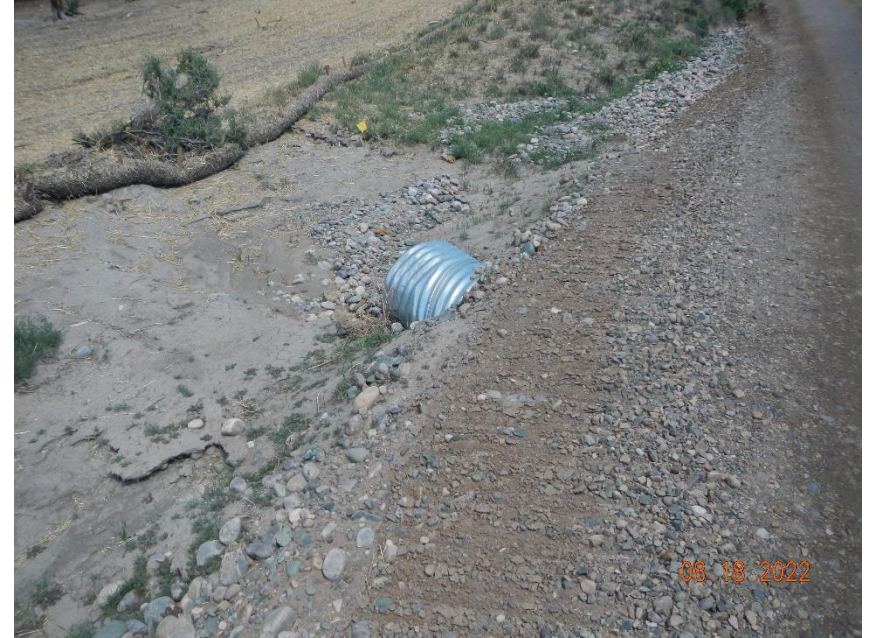
Erosion at culvert on access not inlet protection
