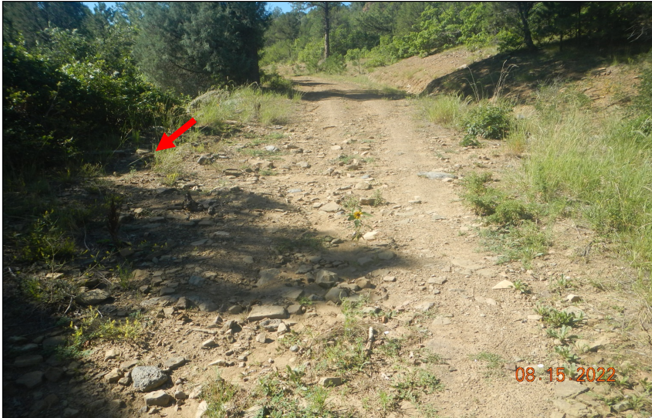
Photo 1. Facing south along the access road. There is a culvert that is filled in with sediment causing stormwater to flow down the road causing erosion. Lat/Long:37.08200, -104.51180.
