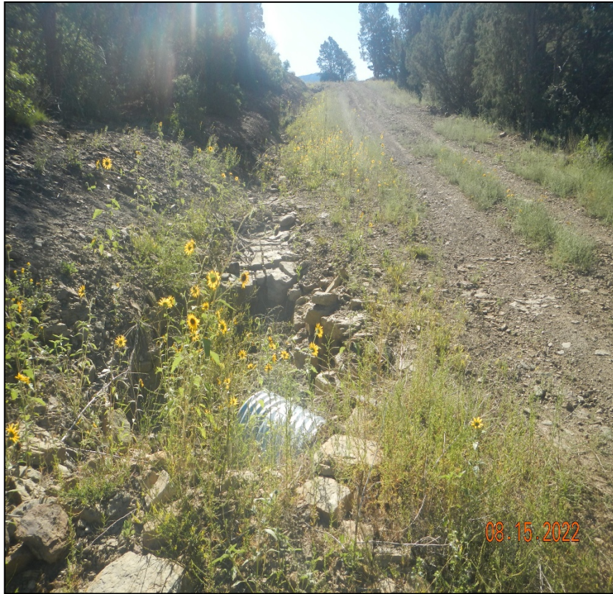
Photo 6. There are culverts installed along the road ascending this hillside.
