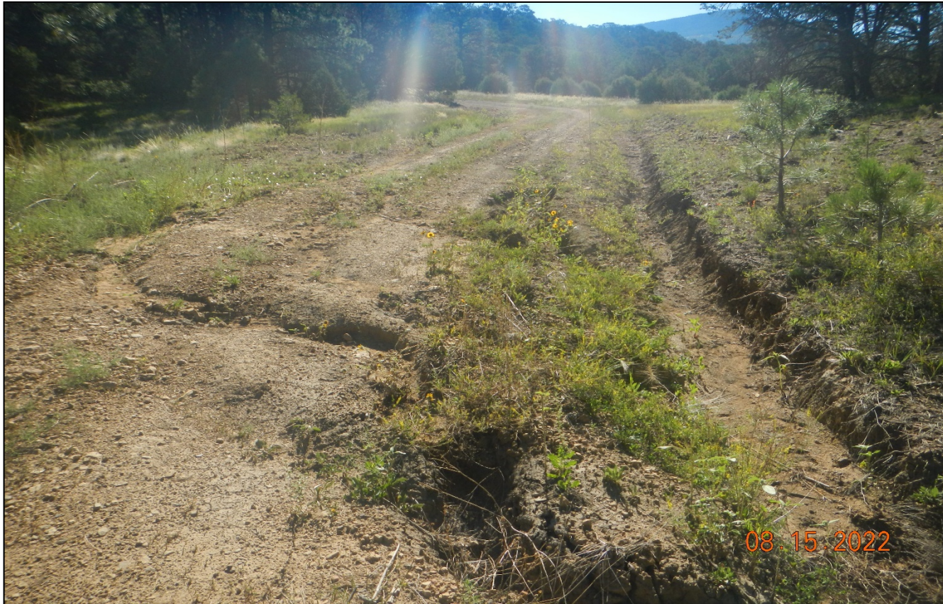
Photo 9. Facing east along the access road. There is erosion of the road in this area that needs to be repaired. There are stormwater divers further up the road that have filled in with sediment causing stormwater to flow down the road to this area. Lat/Long:37.07559,-104.50439
