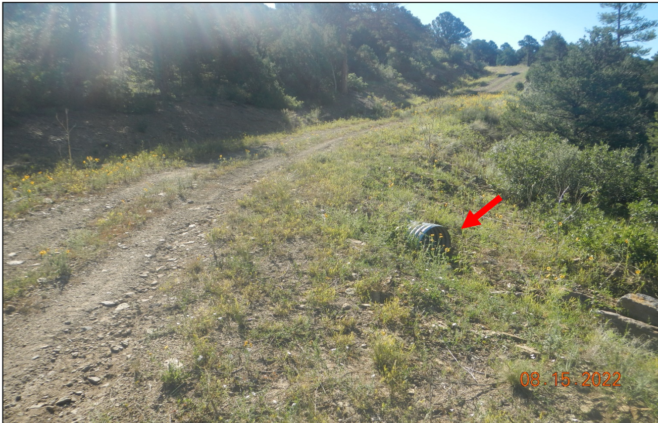
Photo 5. Facing southeast along the road. There are culverts installed along the road. The culvert outlet shown at red arrow has rip/rap outlet protection.
