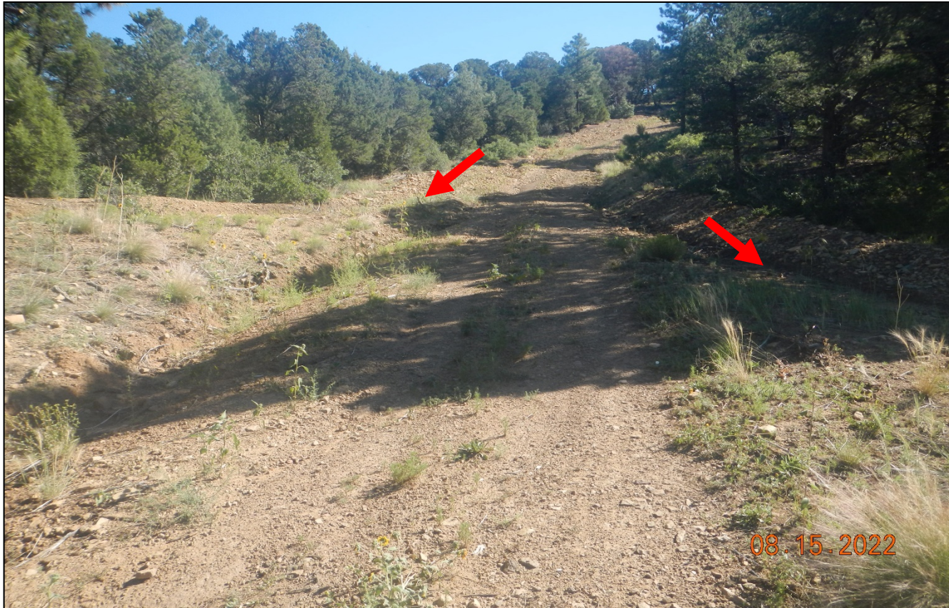
Photo 10. Facing northeast along the access road ascending the hill. The stormwater diversions in this area (red arrows) have filled in with sediment causing stormwater to flow back onto and down the road causing erosion shown in previous photo. Lat/Long:37.07585,-104.50347
