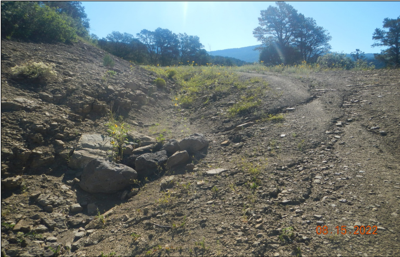
Photo 8. This rock check dam at the curve need to be installed from side to side so stormwater does not flow around the check dam. Lat/Long:37.07425,-104.50717
