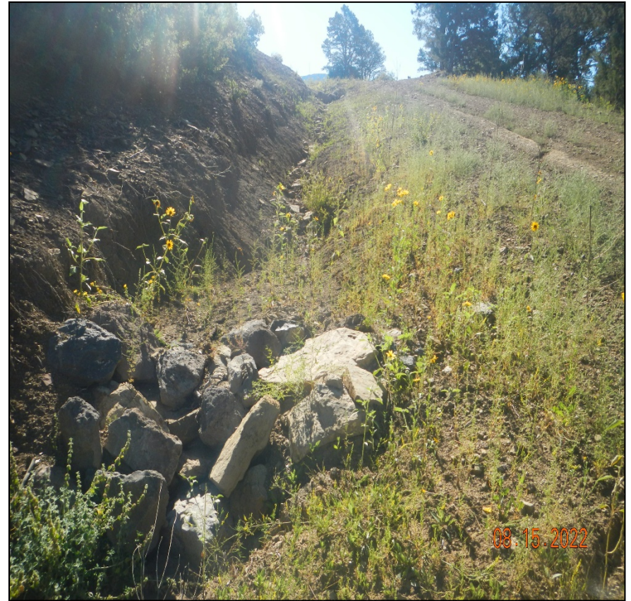
Photo 7. There are multiple rock rip/rap check dams installed along the roadside.
