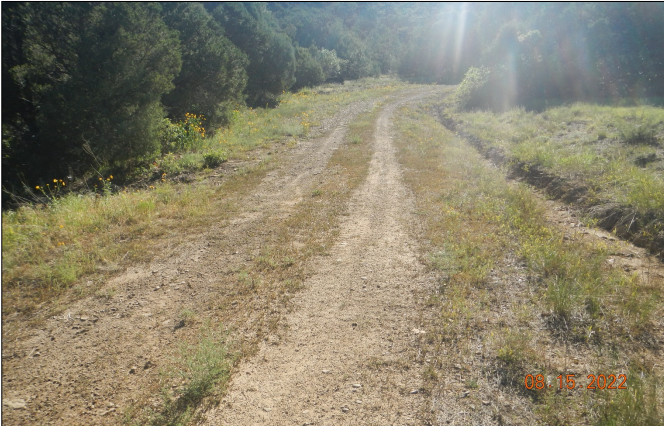
Photo 4. This runoff ditch was not properly installed. The disturbance along the side of the road will need to be seeded and stabilized.
