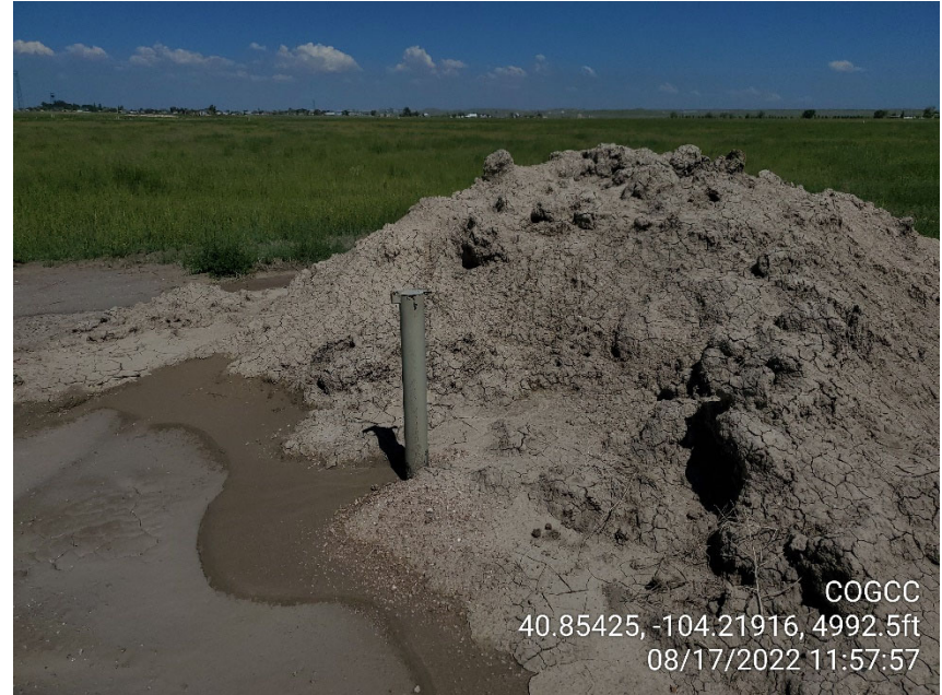
Monitoring well installed at location
