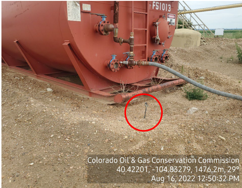
Photo 11: Tank grounded
