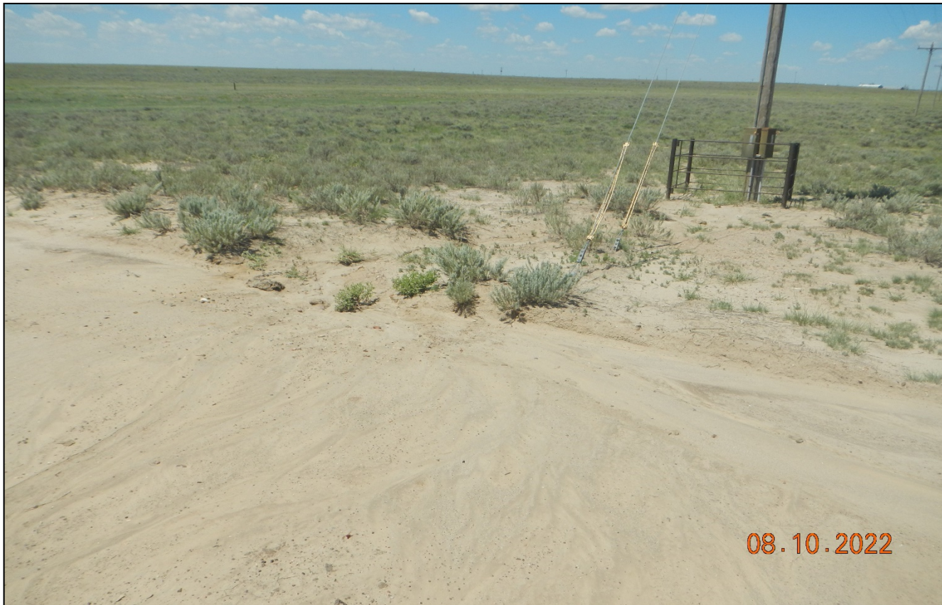
Photo 6. There are signs of sediment movement offsite. BMP's need to be installed.
