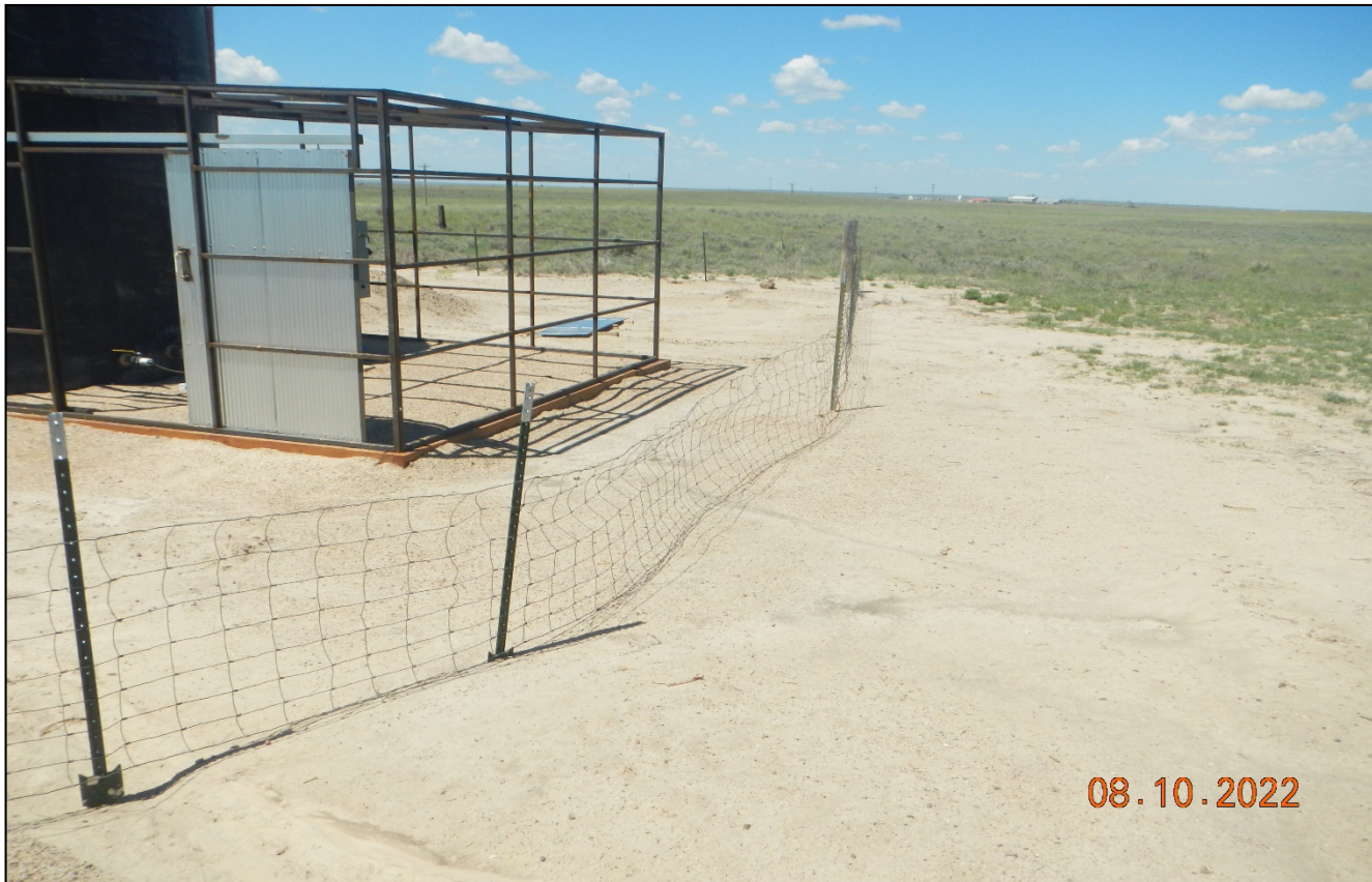
Photo 3. The fence at the tank battery is inadequate and needs maintenance.
