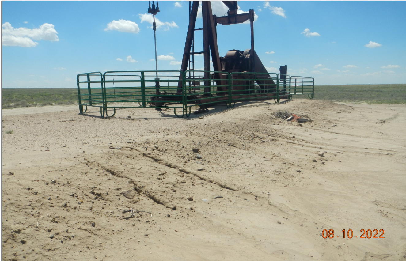
Photo 5. Facing toward the pumpjack. There is stormwater runoff transporting sediment offsite.
