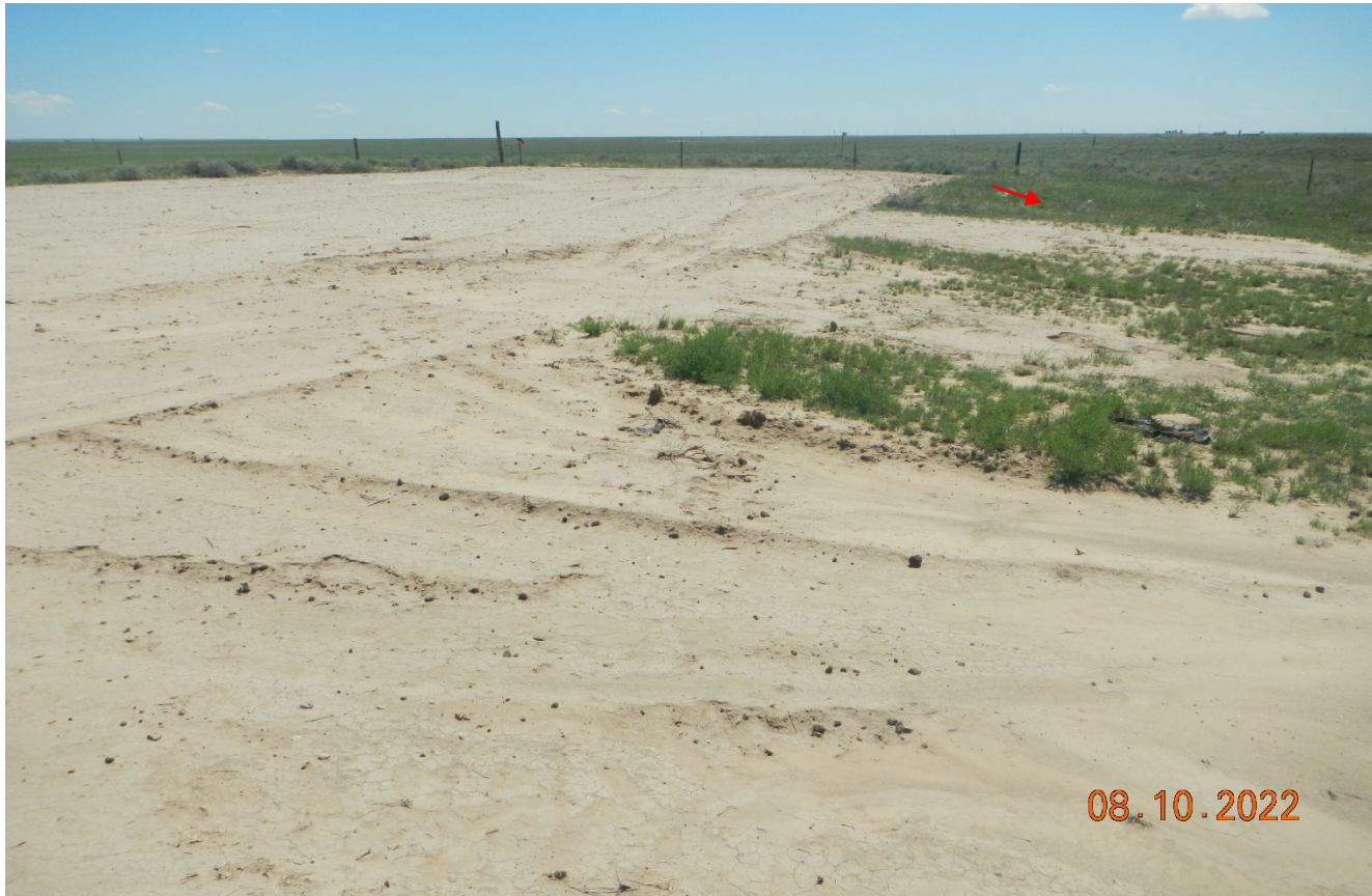
Photo 4. Facing south at the recontoured battery site. There are no stormwater controls installed down gradient and bare soils are susceptible to erosion.
