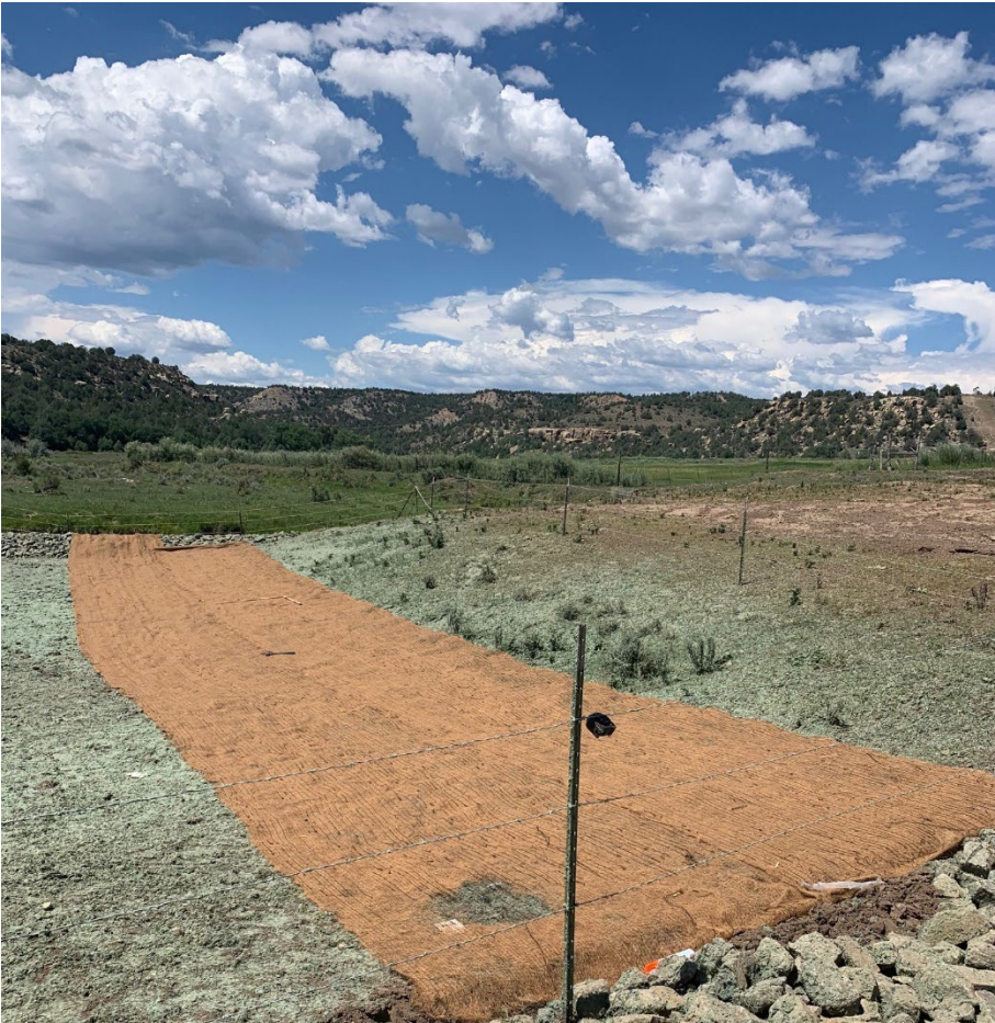
PHOTO 27 Erosion Blanket
