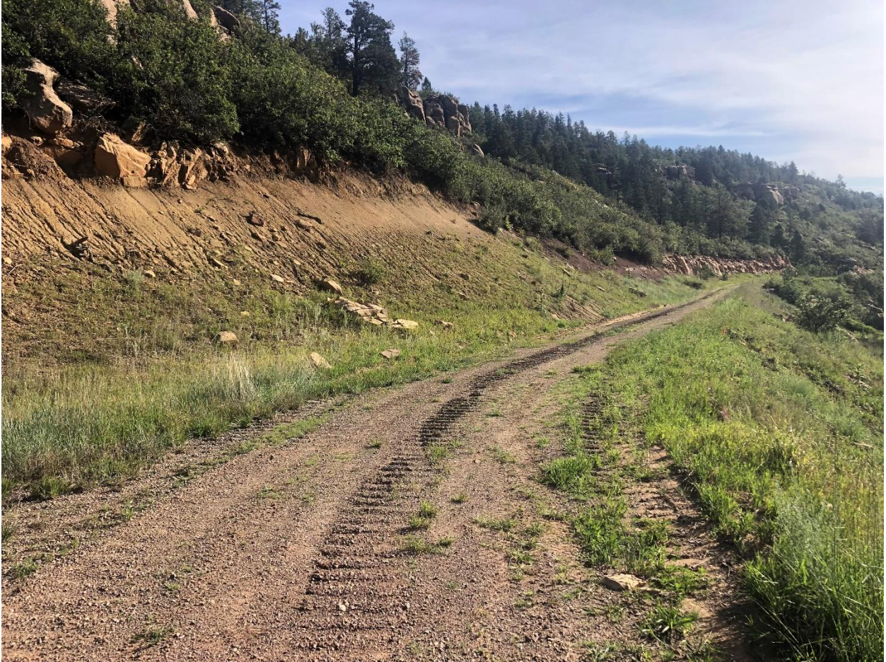
Culverts cleaned rocks removed and recontoured per Rule 1002.f.(2)
