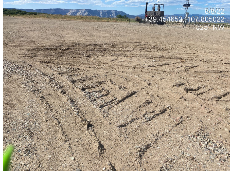
Photo 4. Photo shows control measures to protect and stabilize the production areas remain missing or insufficient at the east of the Location.
