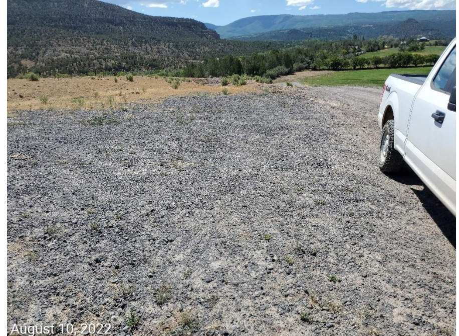
Photo 1: Photos show southern areas of the Location that have not been reclaimed in accordance with 1004 Rules; gravel has not been removed, and areas have not been decompacted, recontoured/regraded and revegetated.
