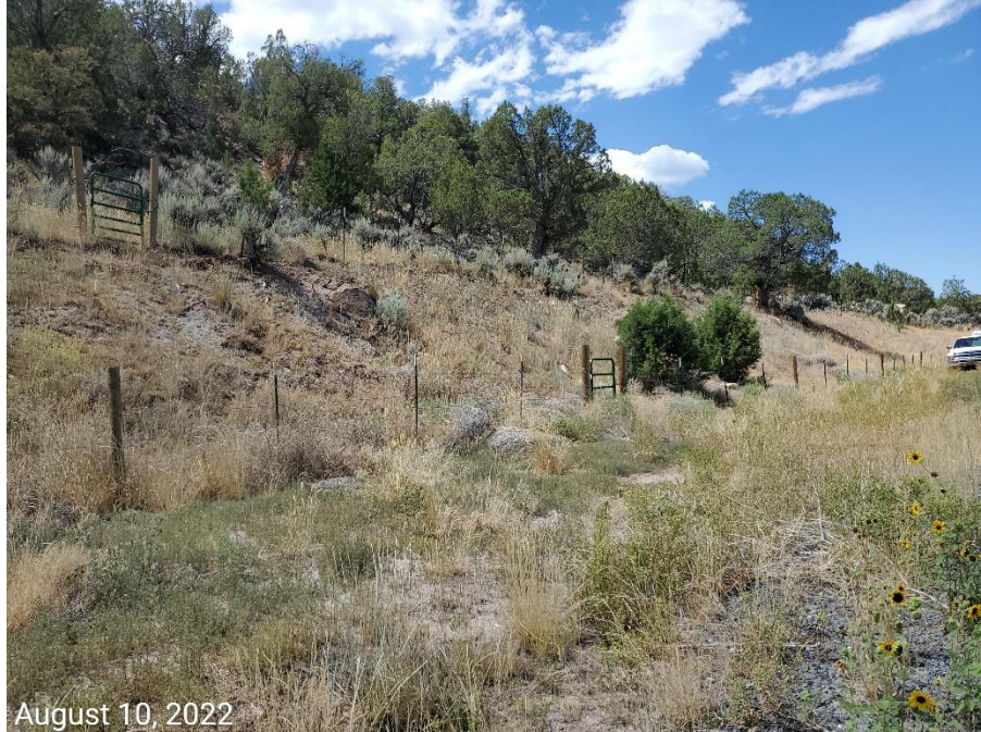
Photo 2: Photos show cut and fill slopes of the Location; location has not been recontoured/regraded.
