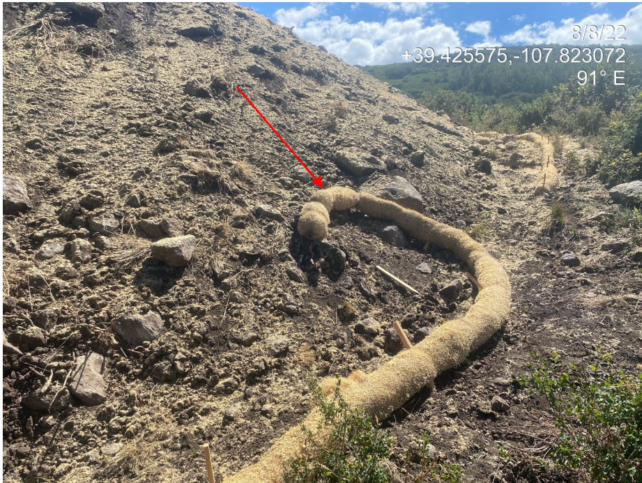
Photo 6. Photo taken from the south shows a straw wattle installed around the perimeter of the topsoil stockpile is in disrepair and is not in proper functioning condition to protect the stockpile. Downslope sections of the wattle were not trenched and backfilled.
