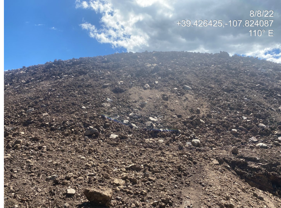
Photo 11. Photo taken from the west of the Location shows soils of the fill slope are unstabilized. Upon completion of construction, slopes must be stabilized.
