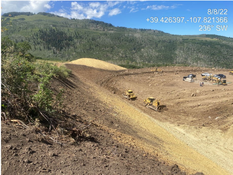
Photo 2. Photo taken from the east shows an overview of the western portion of the Location. Photo also shows the cut slope is unstabilized. Upon completion of construction, slopes must be stabilized.
