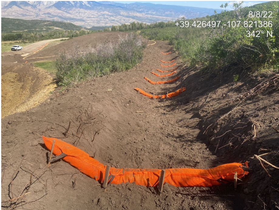
Photo 8. Photo taken from the east of the Location shows the perimeter stormwater diversion ditch. The channel shape has been properly constructed however, soil in the ditch is loose and unconsolidated, acting as a pollutant source. Velocity checks have been installed within the ditch.
