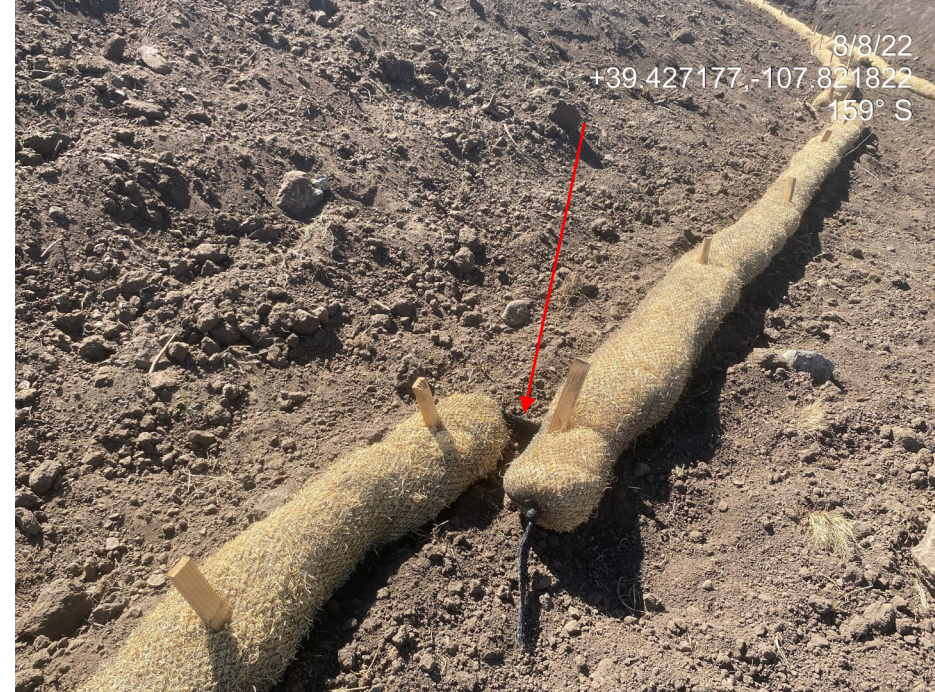
Photo 5. Photo taken from the northeast shows a straw wattle installed around the perimeter of the topsoil stockpile. Adjacent wattles have not been properly installed and wattles have not been trenched and backfilled.
