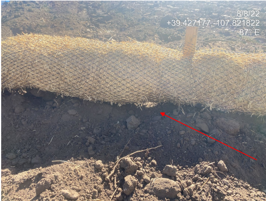
Photo 4. Photo taken from the northeast shows a straw wattle installed around the perimeter of the topsoil stockpile has not been properly installed. The wattle has not been trenched and backfilled.
