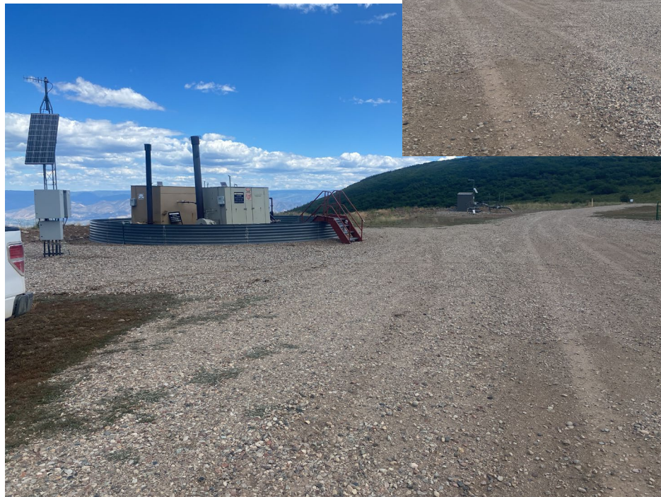
Photo 1. Photos taken from the Location entrance at the west show an overview of the production area. Photos show pad surface has been regraded and gravel applied.
