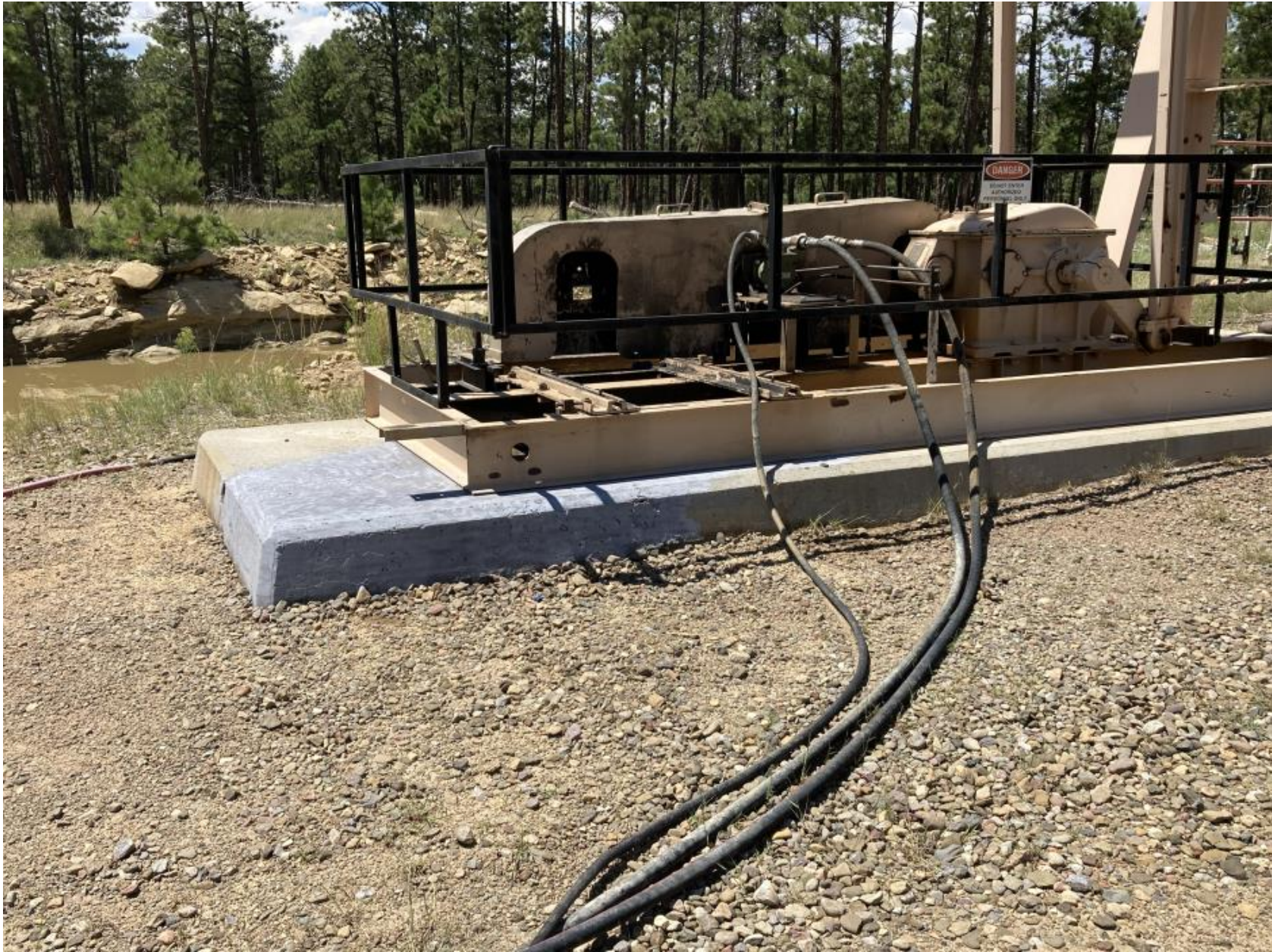
PHOTO 2: MAINTENANCE HAS BEEN PERFORMED, THE IMPACTED SOIL NEAR THE PUMPING UNIT SKID WAS CLEANED UP AND REMOVED FROM LOCATION. THE STAINING ON THE CONCRETE PAD HAS ALSO BEEN REMOVED. THE SELF INSPECTION PROCESS HAS BEEN REVIEWED. CORRECTIVE ACTION COMPLETED 7/1/2022
