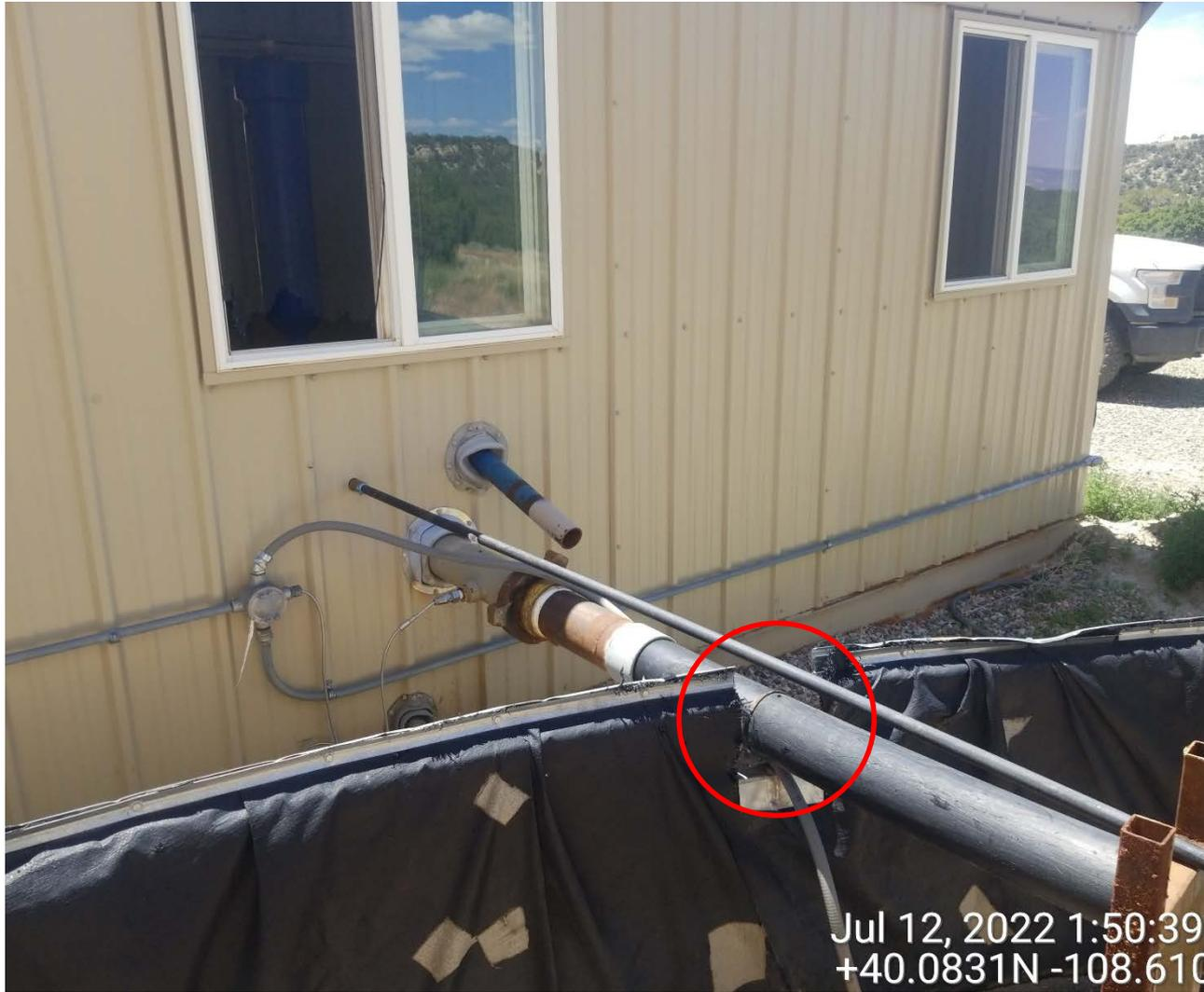
A section of the tank battery secondary containment structure has been removed to accommodate a flowline near the adjacent pump building (red area). Note the various sized patches on the tank battery secondary containment structure.
