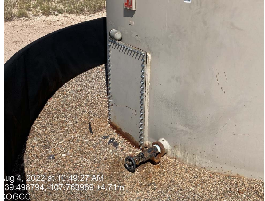
Valve missing cap/plug
