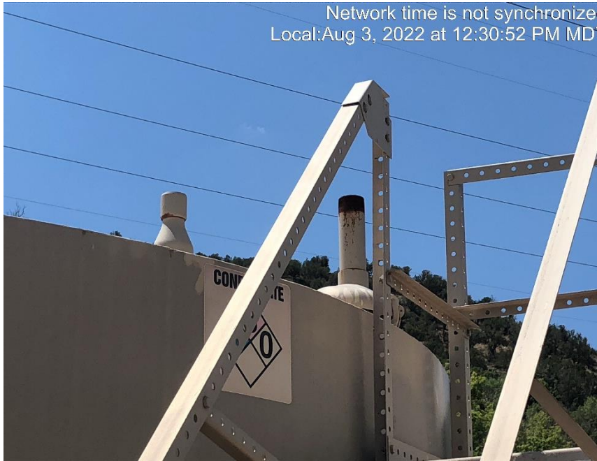
Photo #7418 Vent pipes on tank open ended.
